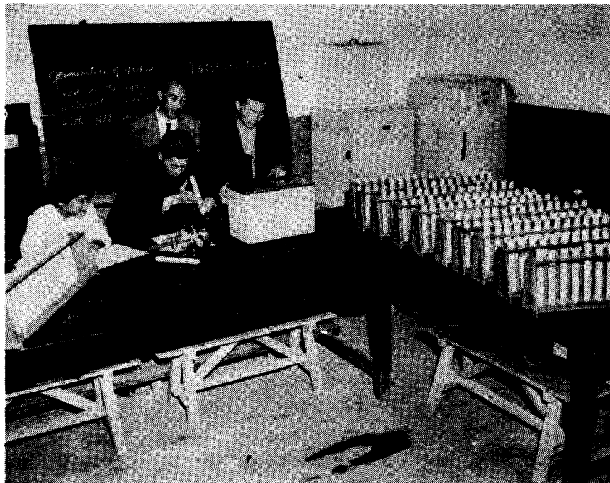
Testing milled rice samples for moisture content. From left Miss Lee Mi-Soon, Prof. Lee Eun-Woong, Chun Cha-Fun (at scale), Lee Han-Sik (reading the meter).
