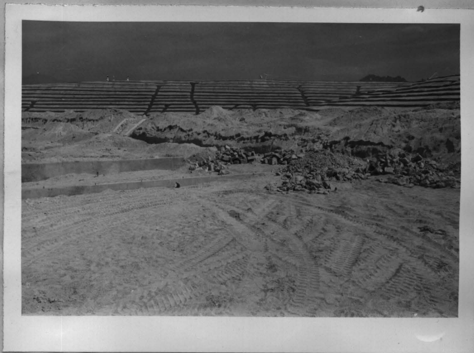
Fig. 6 - Terracing For Erosion Control. Looking North.
