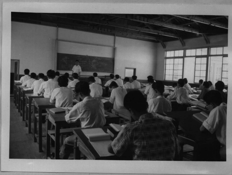
Fig. 9 - Classroom in Repaired Building. (See Fig. 2, Building "C".)
