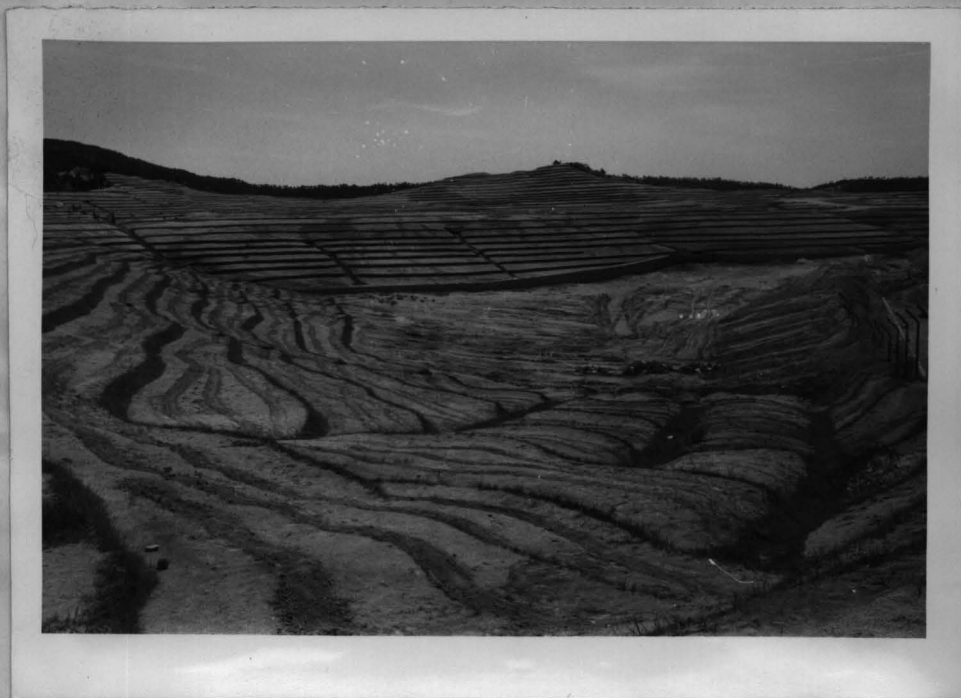
Fig. 7 - Terraces For Erosion Control. Upper Level. Looking East.
