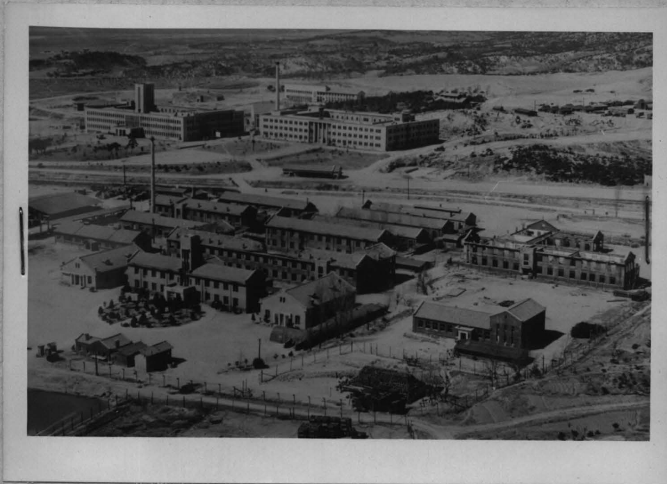
Fig. 1 - College of Engineering - Damaged Mining Compound in Foreground.
