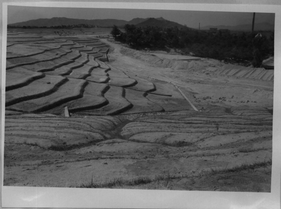
Fig. 8 - Terraces For Erosion Control. Lower Level. Looking South. (See Fig. 5)
