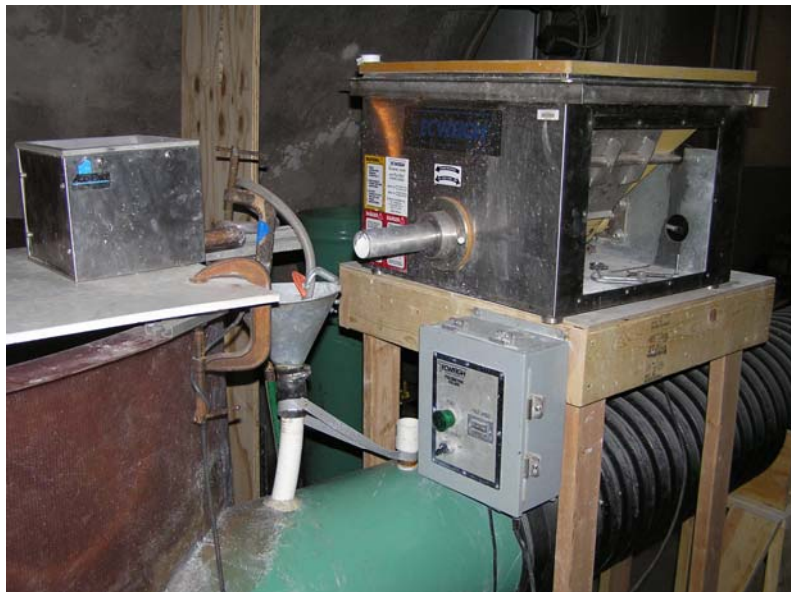
Figure 2.3. Two sediment feeders were located on the inflow pipe upstream of the M_1 manhole. Clay particles were separately to avoid any coagulation of particles before entering the influent pipe.
