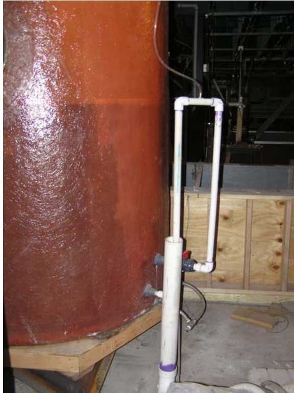
Figure 3.4. Draining system of the manholes
