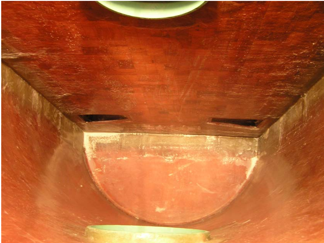
Figure 1.2. View of the baffle wall from the second compartment of the M_2 manhole.
