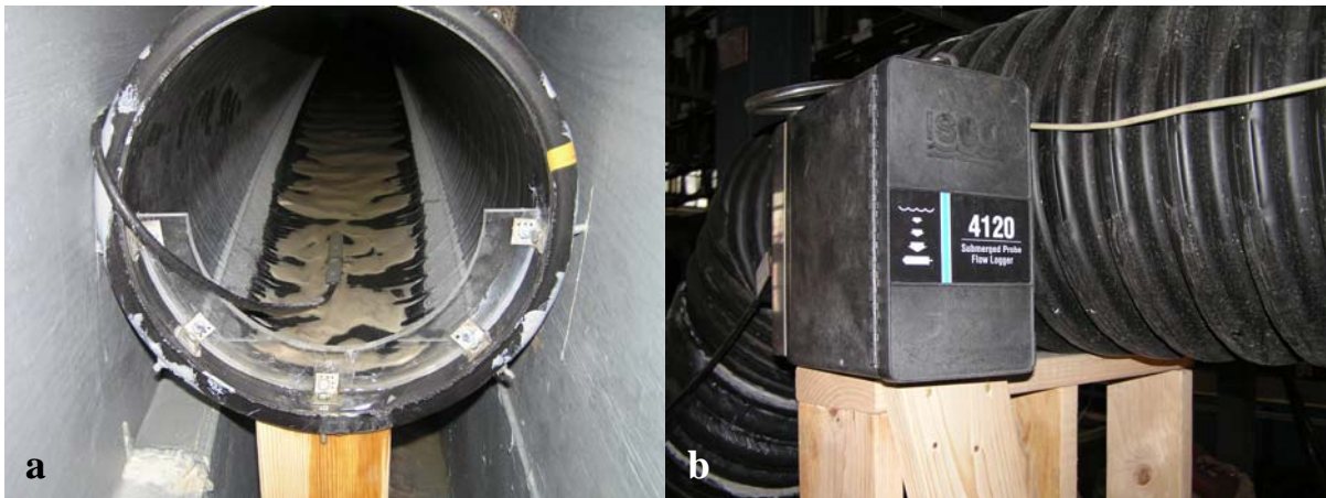
Figure 2.2. (a) The circular weir and submerged pressure transducer probe in the outflow pipe, and (b) an ISCO 4120 data logger to record the flow data.
