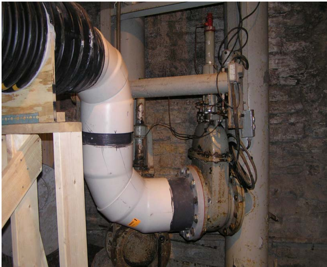
Figure 2.1. The 12-inch supply pipe, the 12-inch gate valve, and the 12-inch PVC to 15-inch HDPE pipe expansion for the inflow pipe.
