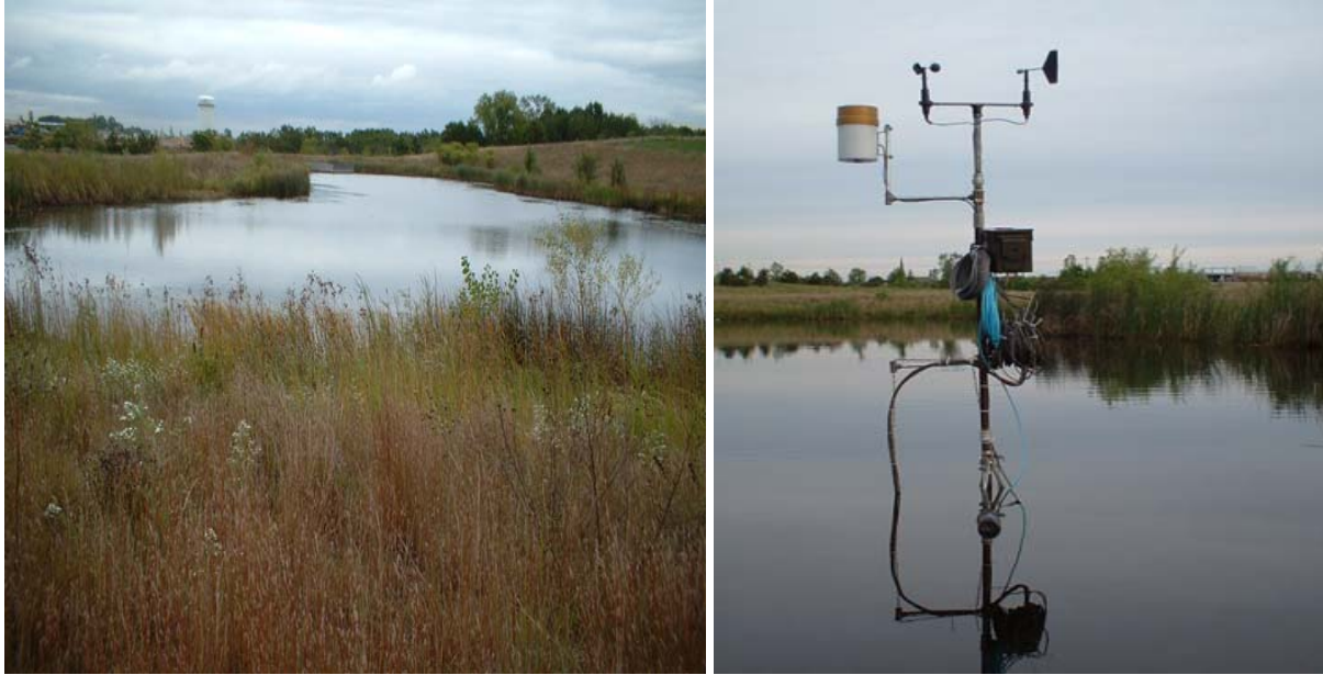
Figure 5.2 Ground level photograph of the State Farm stormwater detention pond, viewed from west to east, and close-up of the measurement station installed in the pond.
