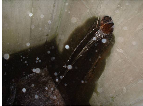
Figures 6.2.6 – 6.2.7 Overflow weir (left panel) and circular 0.203m (8”) diameter outlet (right panel) at East end of pond where Vemco temperature logger was placed.
