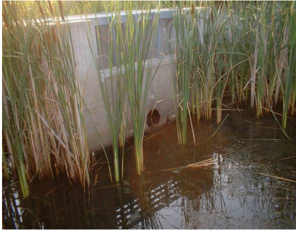
Figures 6.2.6 – 6.2.7 Overflow weir (left panel) and circular 0.203m (8”) diameter outlet (right panel) at East end of pond where Vemco temperature logger was placed.
