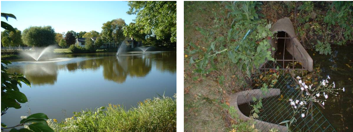
Figures 4.3.1 – 4.3.4 Highland Court Pond (Index # 66-03). West Marsh Drainage Area.
