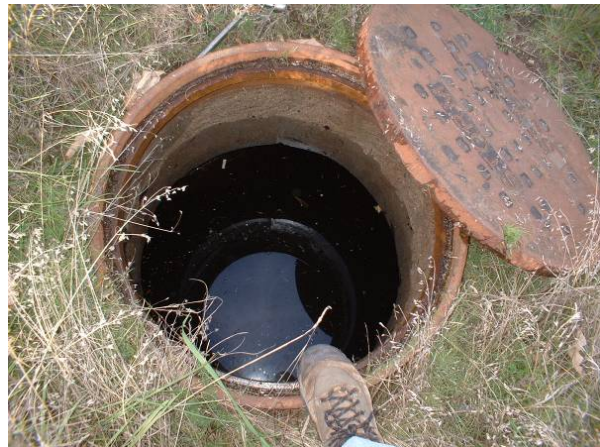
Figures 6.2.4 – 6.2.5 Manhole of single stormsewer draining into the pond at West end, where a Vemco temperature logger was placed.
