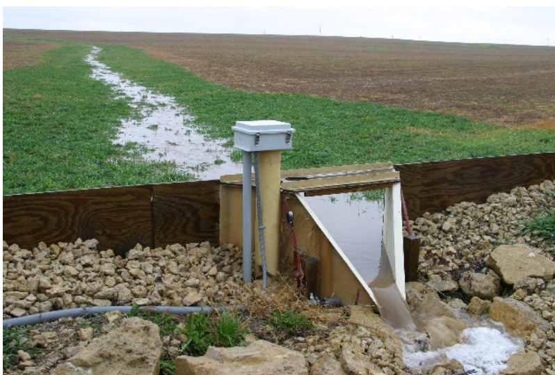
Figure 3. H Flume without approach section. (Photo by Dennis Busch).
