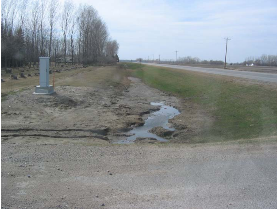
Figure 17. Deposition of sediment in roadside ditch.
