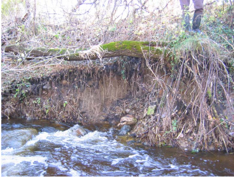
Figure 9. Bank erosion within deep, narrow section of Hay Creek where channel cuts through glacial till. Note large cobbles on banks and stabilizing bed. The incised stream reach is approximately 1 km long. Photo taken at approximately point X in Figure 4.
