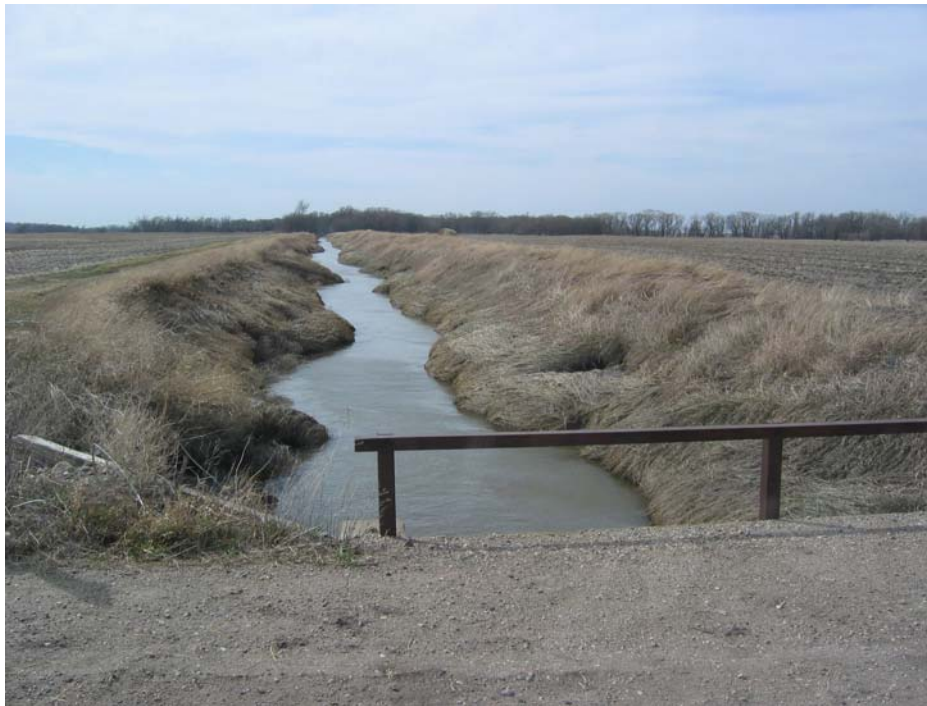
Figure 8. Bank erosion on straightened portion of Hay Creek. Photo taken upstream from point M in Figure 4.
