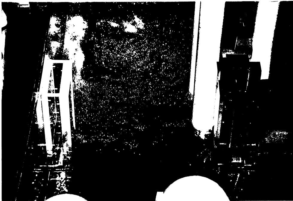
Fig. VIII-5. Air from blowout surfacing in pump sump. Withdrawal rate of 30,000 gpm through screen being cleaned.
