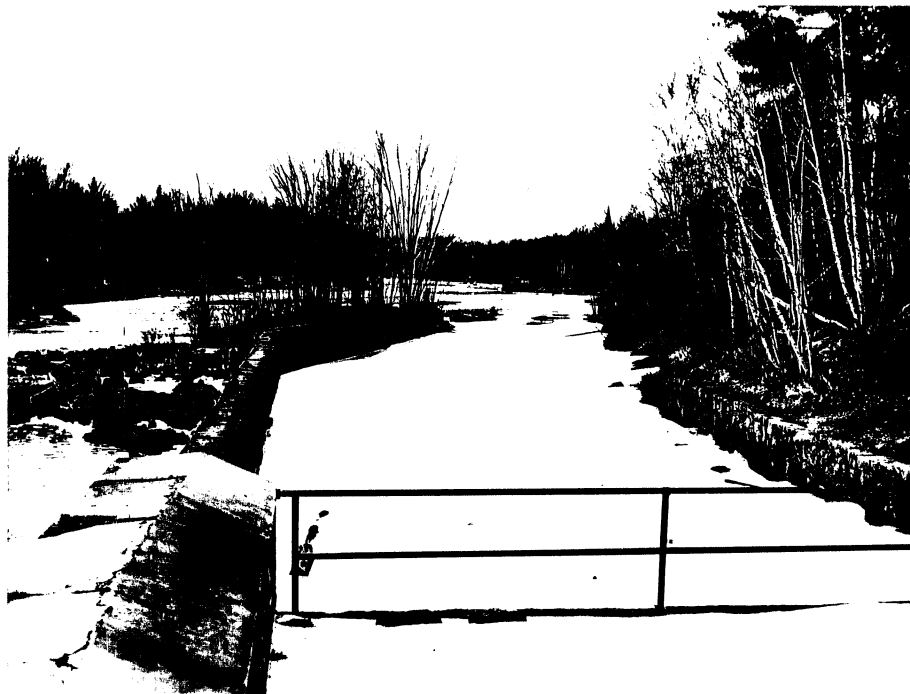
Fig. 4b. Photograph of Tailrace and Downstream Stream Reach from Generator Room. Kettle River Dam, February 19, 1981.
