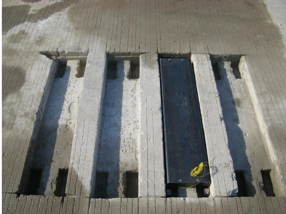
Figure 10: WIM Sensor Installed in a Slot at MnROAD
