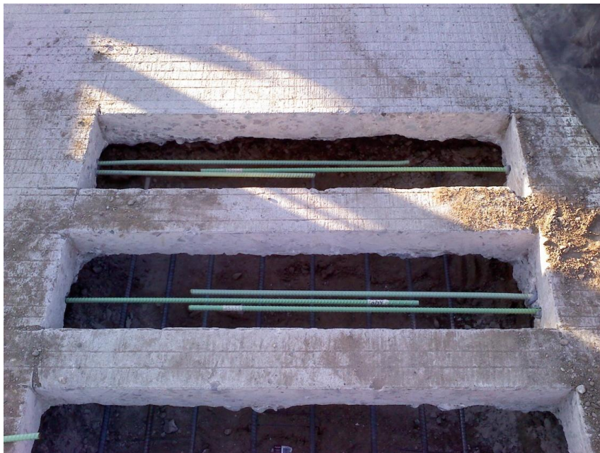
Figure 50: Rebar was used to form a bond between the new and old forms
