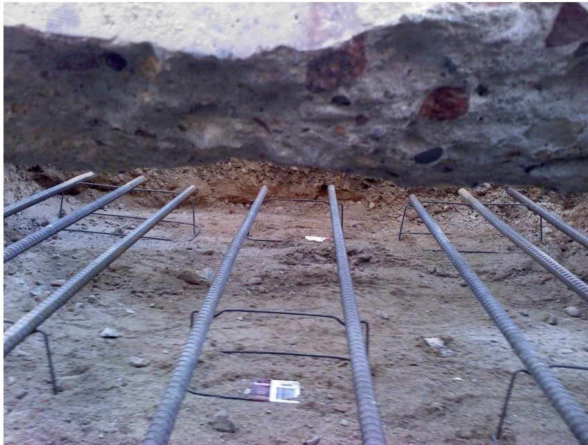
Figure 49: Rebar was placed in the hole before pouring to strengthen the new sub base.
