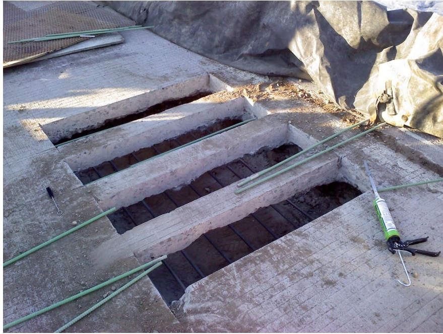
Figure 48: Holes were cut into the concrete and material removed from below the road.
