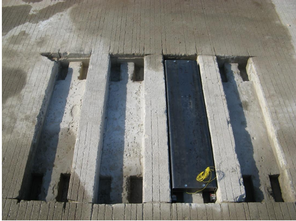
Figure 51: Once the new sub base was poured, the sensors could be installed
