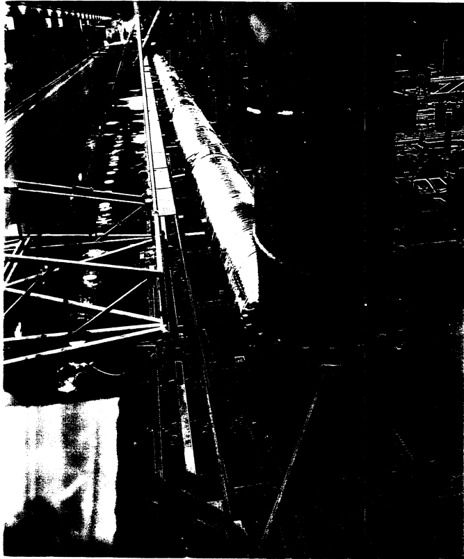
Fig. 8 - Looking Downstream at the Experimental Arrangement with 24 in. Pipe Installed
