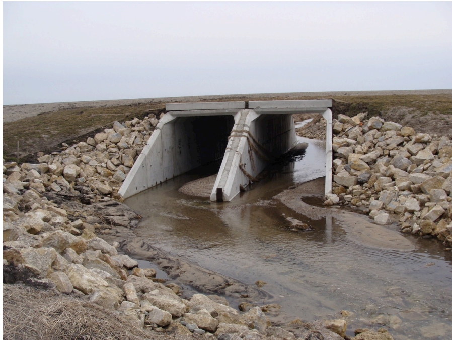
Figure 57. View of the Double-Box Culvert Beneath Mower County Highway 6 (Looking Downstream). March 24 th , 2010.
