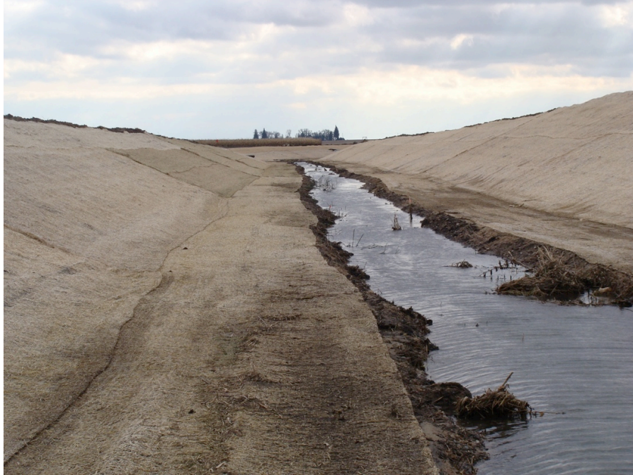
Figure 51. A View of the Channel Looking Downstream from the Field Road Crossing. November 4 th , 2009. Photo by Brad Hansen.
