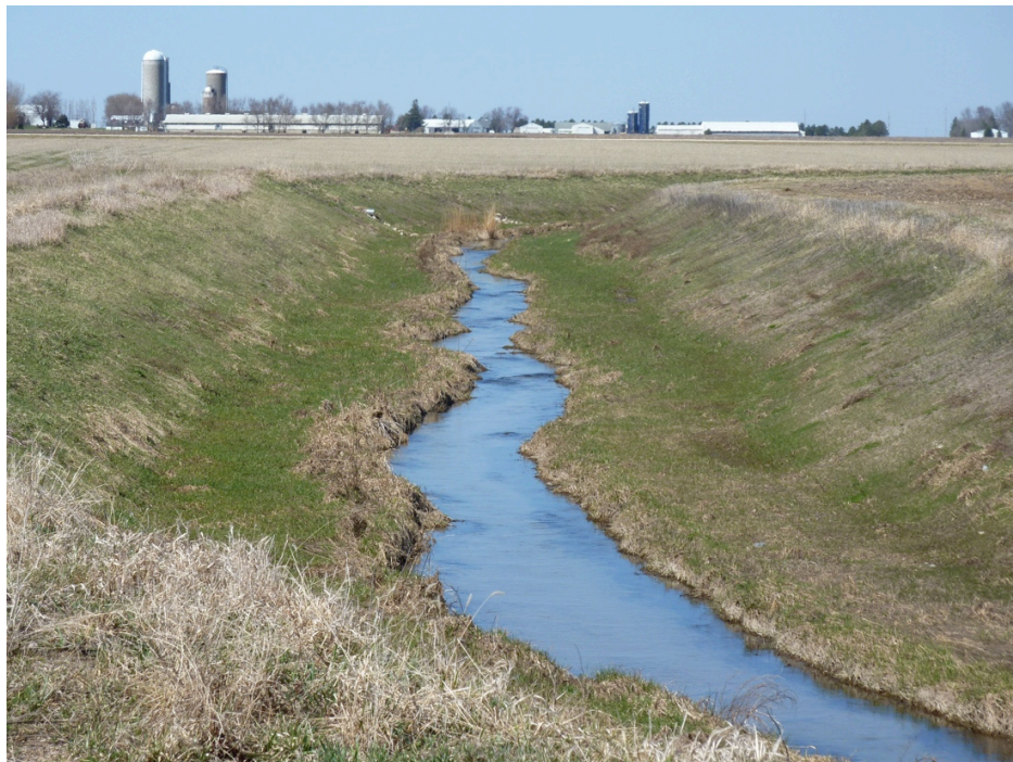
Figure 68. A View Looking Upstream from 24+00. April 12 th , 2011.
