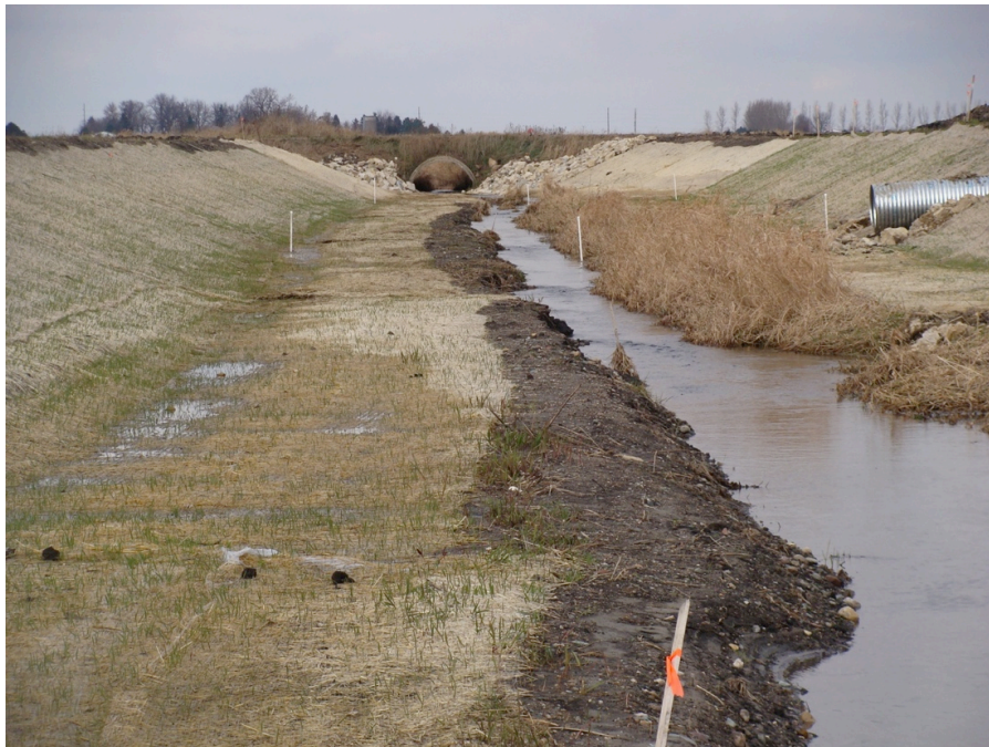
Figure 52. A View of the Upstream End of the Ditch, Taken Looking Upstream from 6+00. The Vegetation Emerging Through the Erosion Control Mat Shows the Approximate Extent to which Vegetation Emerged in 2009. November 4 th , 2009. Photo by Brad Hansen.
