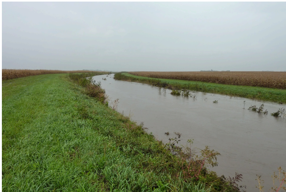
Figure 63. View of the Mullenbach Two-Stage Drainage Ditch During a High-Flow Event on September 23 rd , 2010. Picture Taken Looking North from Just North of Mower County Highway 6.
