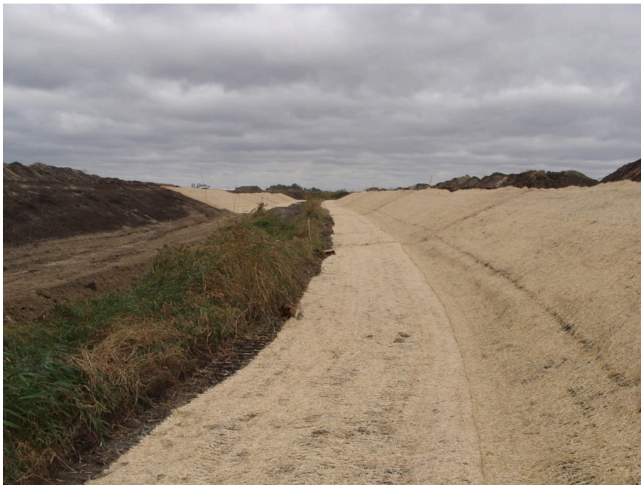
Figure 46. Erosion Control Mat Covering the Ditch Benches and Banks at the Upstream End. Photo Taken Looking Upstream from Approximately 10+00. September 28 th , 2009. Photo by Brad Hansen.
