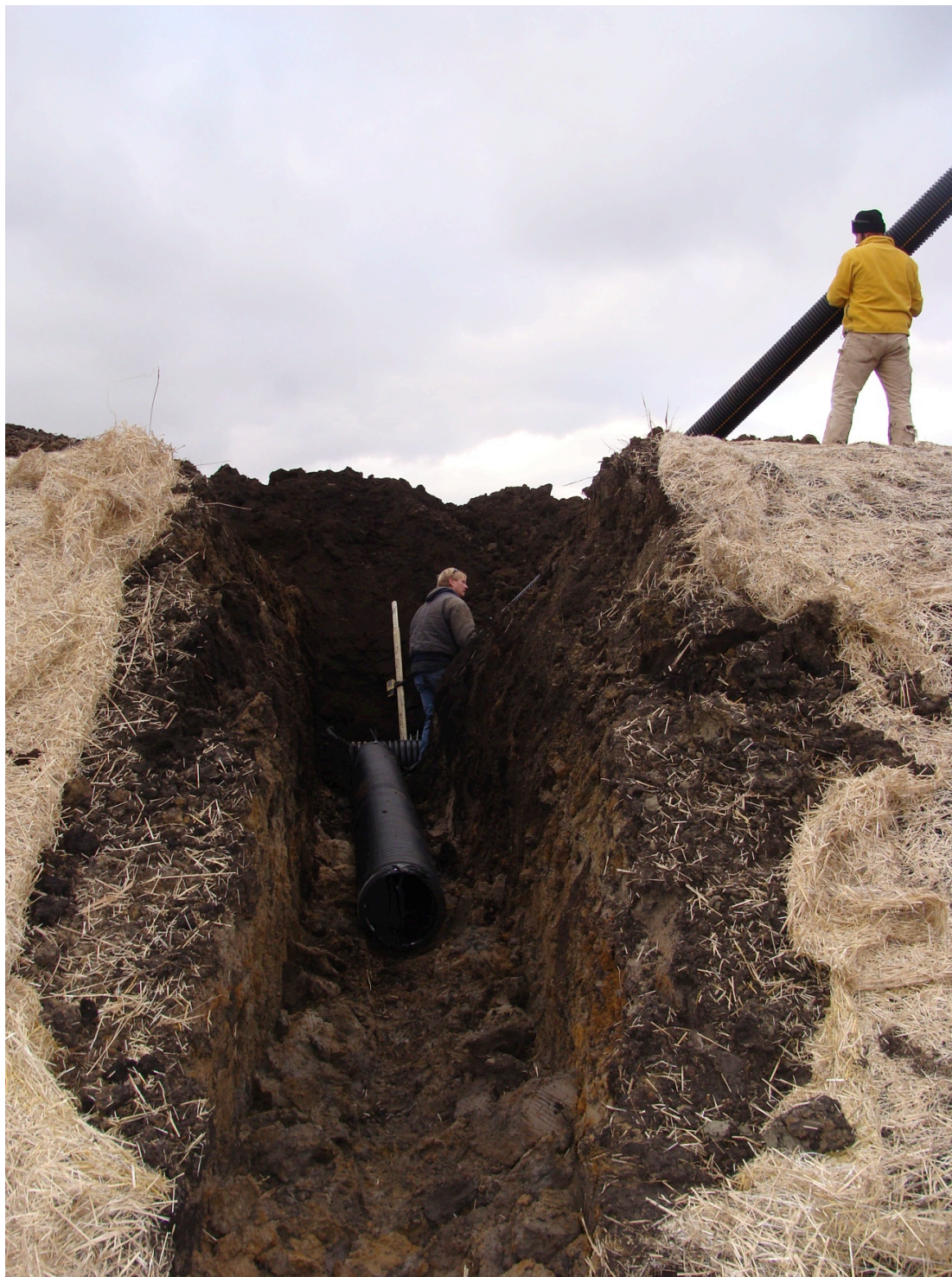
Figure 54. The First Section of Seepage Trench Outlet Pipe (12" Plastic) Exiting the Seepage Trench Toward the Channel. November 4 th , 2009. Photo by Brad Hansen.
