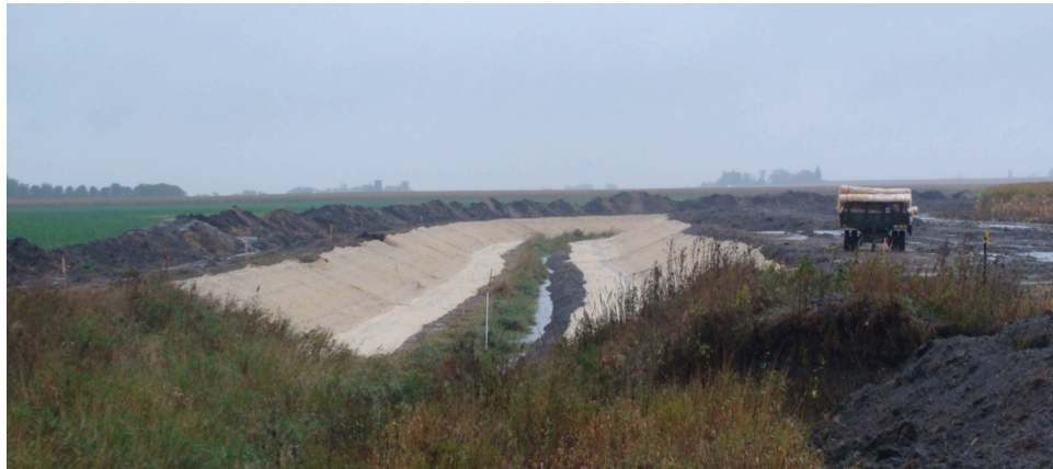
Figure 44. A View of the Completed 2-Stage Channel Form at the Upstream (North) End of the Ditch. Photo Taken Looking Downstream from 120 th Street. October 1 st , 2009. Photo by Brad Hansen.
