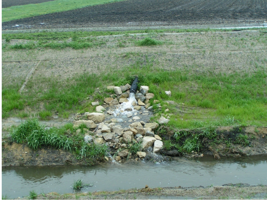
Figure 61. The Tile Outlet at 5+88, with Vegetation Emerging on the Bench and Bank. May 2010.
