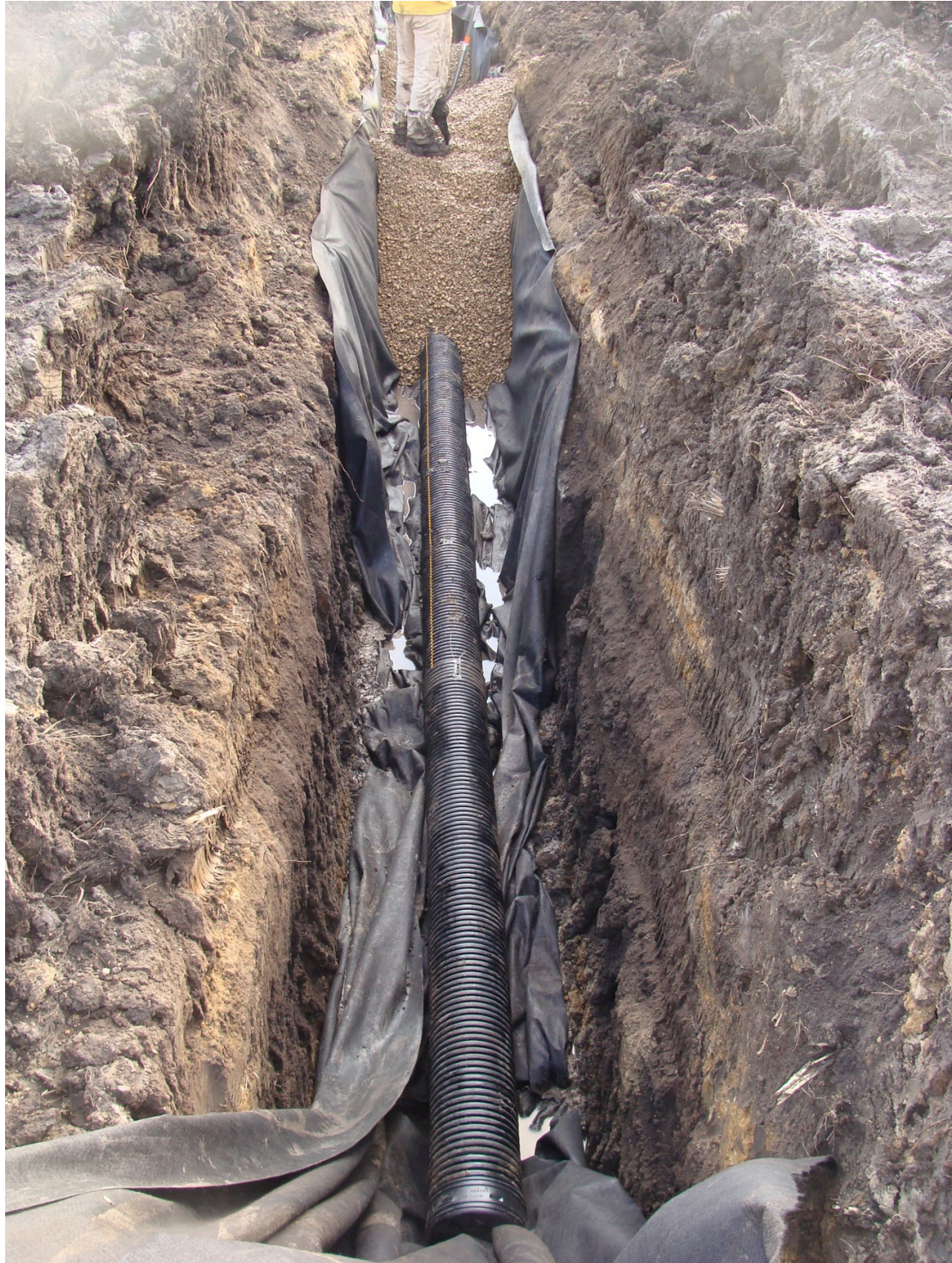
Figure 56. A View of the Longitudinal Drainage Pipe (8" plastic) Installed at the Bottom of the Seepage Trench to Collect Water and Carry it to the Seepage Trench Outlet Pipe. November 4 th , 2009. Photo by Brad Hansen.
