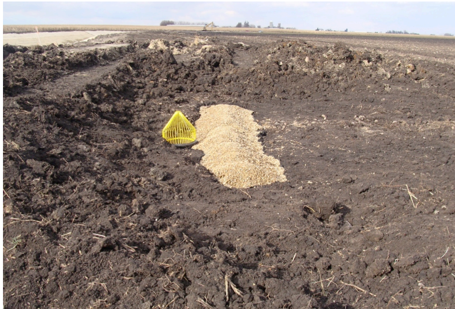
Figure 50. The Rock Trench Side Inlet Intake Structure. Note the Mounded Pea Gravel, which Routes Water Downward into the Rock Trench. The Auxiliary Inlet is to the Left of the Mounded Rock, and Includes a Trash Rack to Prevent Plugging of the System. November 4 th , 2009. Photo by Brad Hansen.
