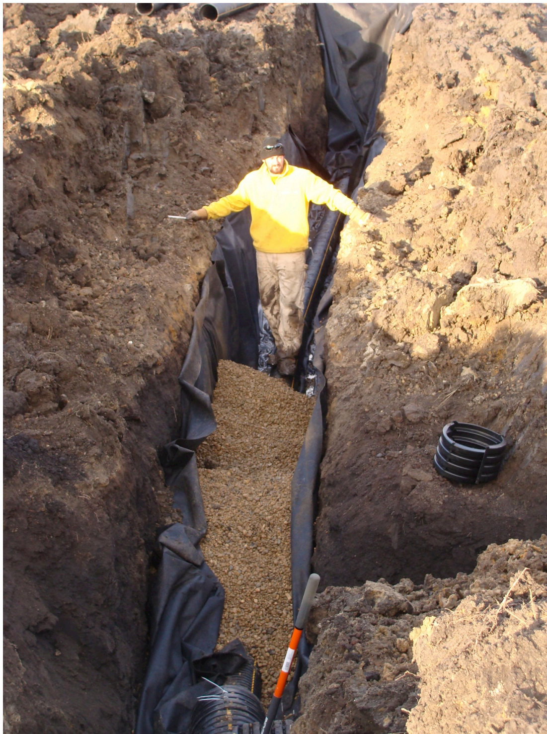
Figure 55. The Seepage Trench Being Filled with Pea Gravel (Note the Liner to Maintain the Gravel Within the Trench). November 4 th , 2009. Photo by Brad Hansen.
