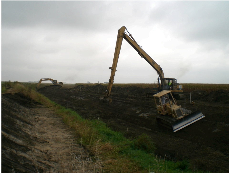
Figure 43. Beginning of Excavation at the Upstream (North) End of the Ditch Reach. Two Backhoes are Excavating the Ditch Benches while the Other Machine is Leveling the Bench and Bank Slope. September 23 rd , 2009.
