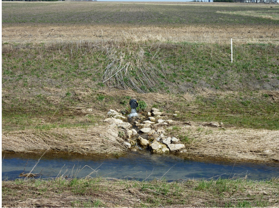
Figure 69. A Tile Outlet and Riprap Reinforcement. April 12 th , 2011.
