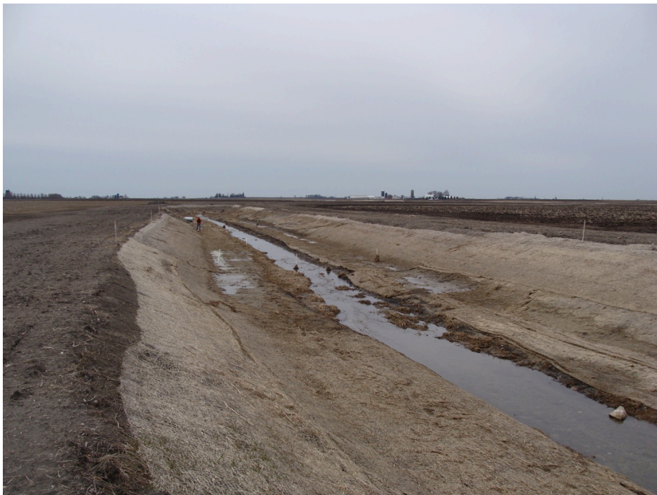
Figure 60. A View of the Upstream Section of Ditch (Taken from 1+00 Looking Downstream). March 24 th , 2010.
