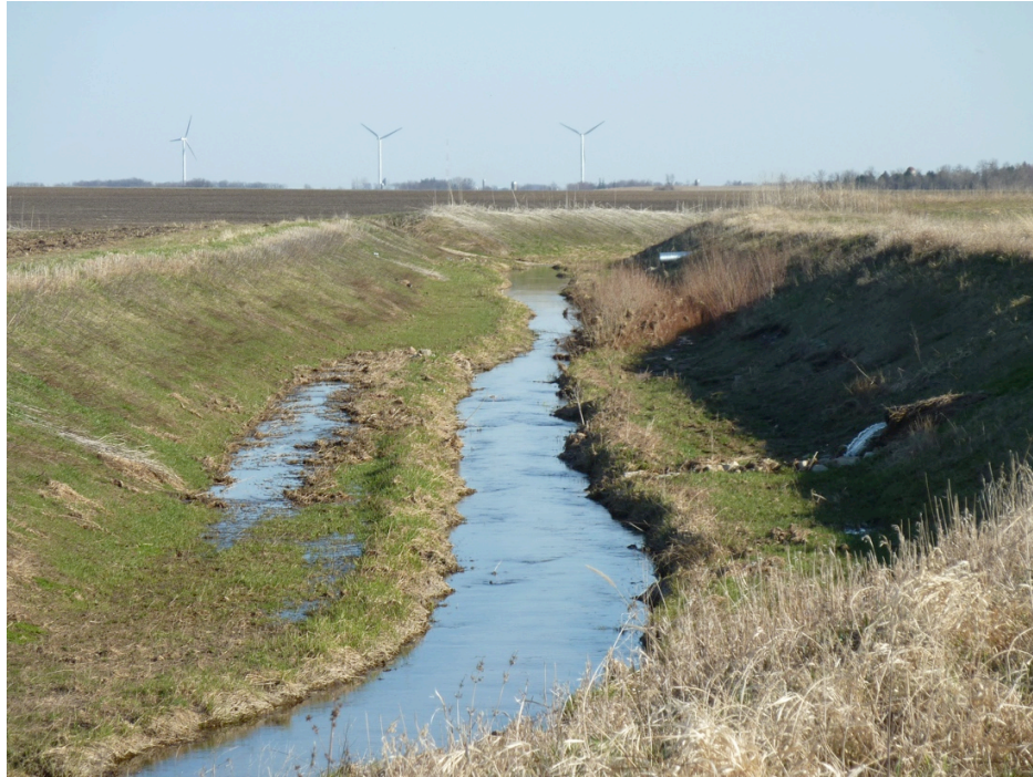
Figure 67. A View of the Channel Looking Downstream from 26+00. The Tile Outlets at 28+00 (Left and Right Banks) Are in the Picture. The Left Bench Includes a Linear Treatment Structure. April 12 th , 2011.
