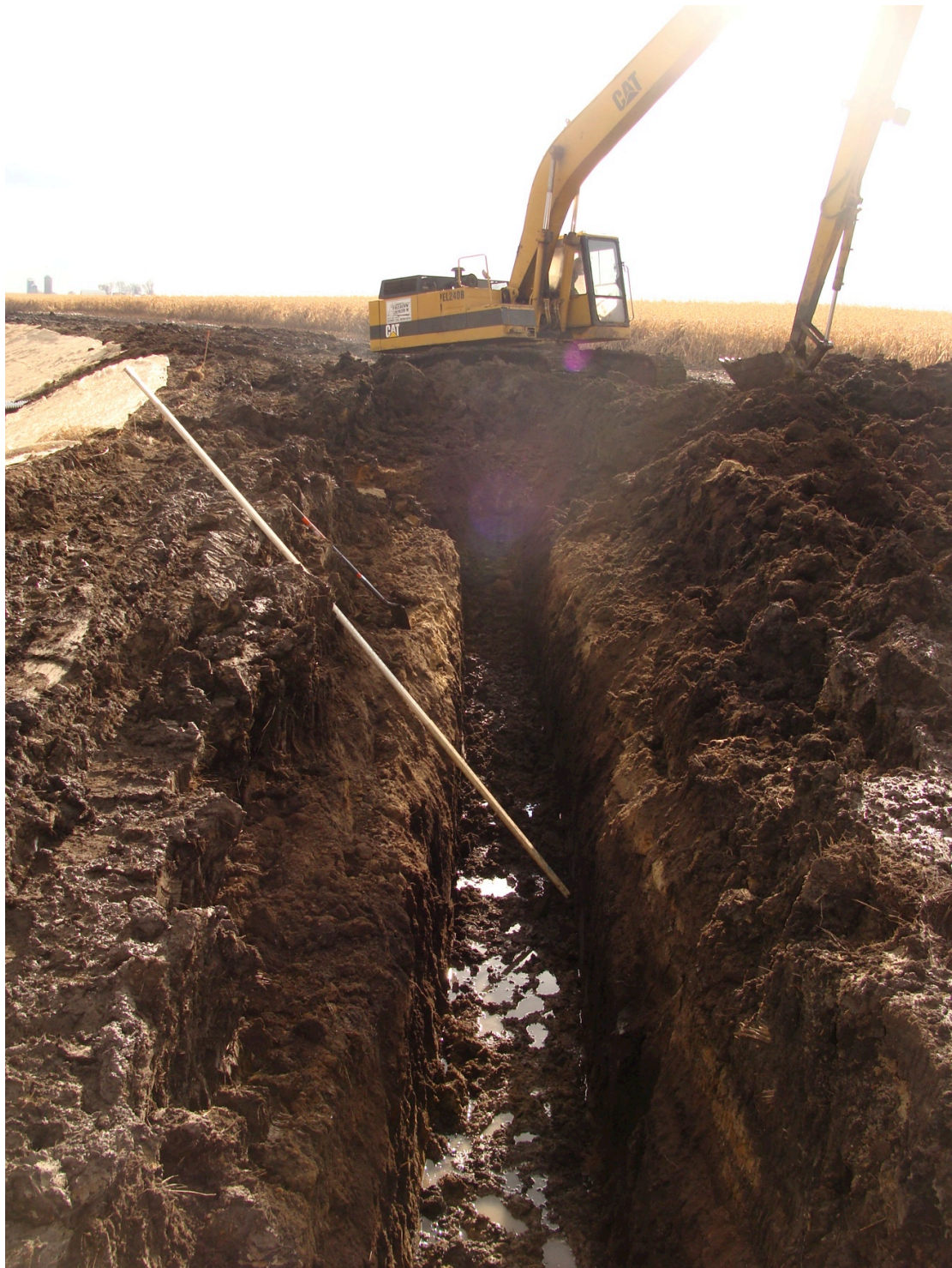
Figure 53. The Excavated Seepage Trench in the Right Bank at 22+00 Before Being Filled. November 4 th , 2009. Photo by Brad Hansen.
