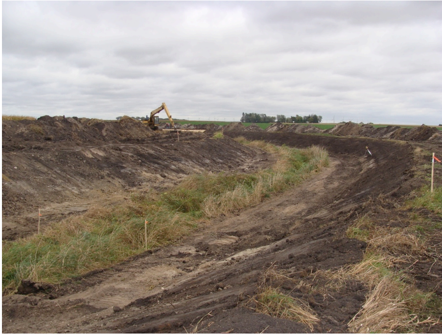
Figure 45. Excavation Continues Through the Bend Near 12+00. Photo Taken Looking Upstream. September 28 th , 2009. Photo by Brad Hansen.
