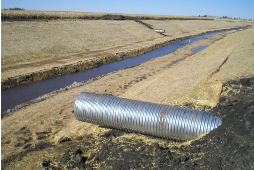
Figure 47. Photo Showing the Side Inlets at 58+28 (Foreground) and 57+00 Following Construction. Note that This Photo was Taken Before Riprap Armoring Was Placed at the Outlets of These Structures. Photo Taken Looking Upstream. November 2 nd , 2009.
