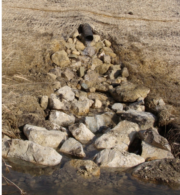
Figure 49. A Tile Outlet Discharging Onto the Ditch Bench After Construction. The Riprap Armoring Protects the Bench from the Erosive Power of the Tile's Discharge. November 4 th , 2009. Photo by Brad Hansen.
