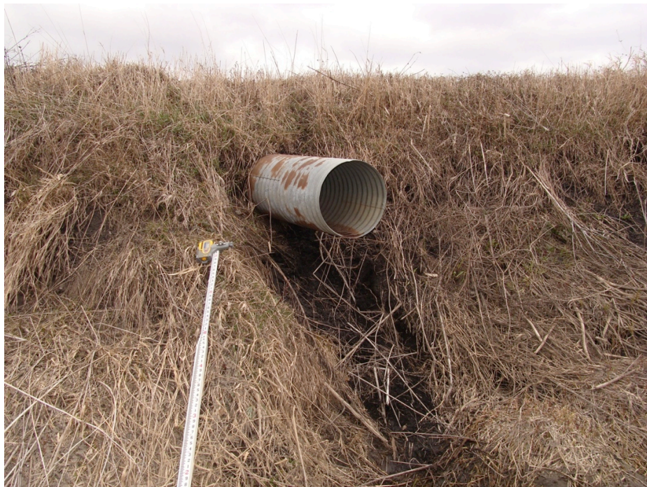
Figure 42. The Side Inlet on the Left Bank at 52+00. March 31 st , 2009. Photo by Brad Hansen.
