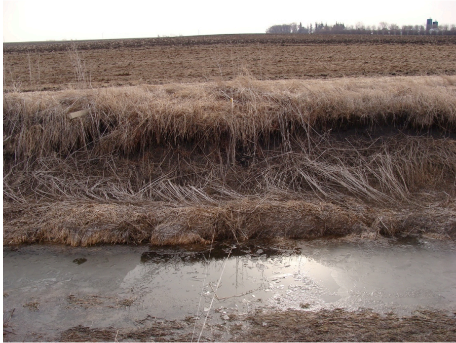
Figure 41. Bank Undercutting and Overhang with a Bench Feature at the 46+54 Cross-Section. March 31 st , 2009. Photo by Brad Hansen.
