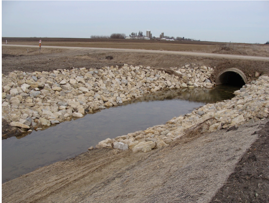
Figure 59. A View of the Culvert Beneath 120 th Street (Looking Upstream). March 24 th , 2010.
