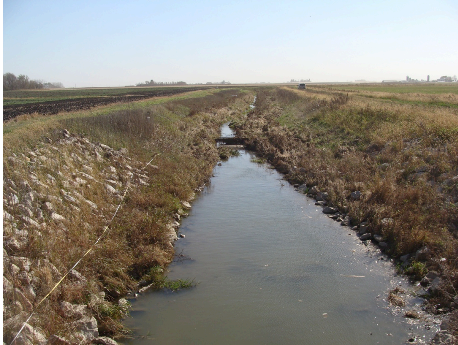
Figure 65. A View of the Channel Looking Downstream from 120 th Street. October 21 st , 2010. Photo by Brad Hansen.
