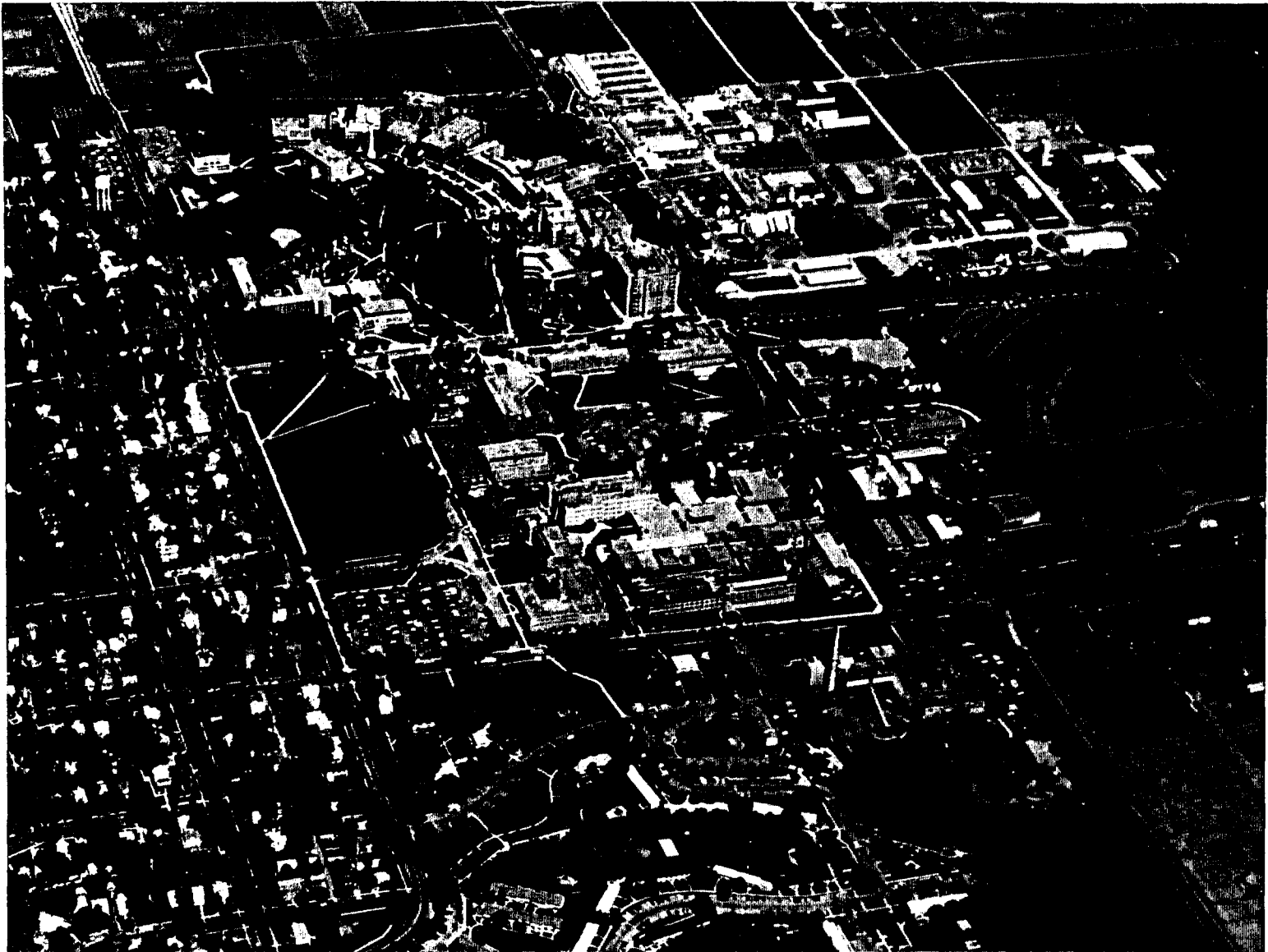
Aerial of existing St. Paul Campus (Source: Saari & Forrai Photography Inc.)
