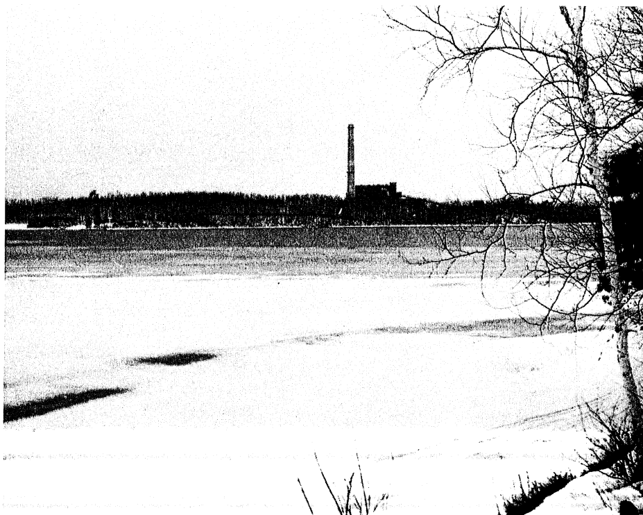
Fig. 17 - View Looking across Colby Lake from Beach Area toward Power Plant - March 2, 1974
