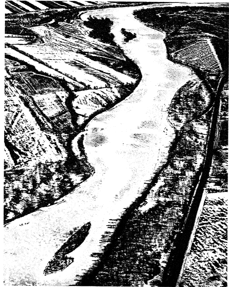
Fig. 5 - Aerial View of Mississippi River Upstream of Sartell, Minnesota - March 10, 1974
