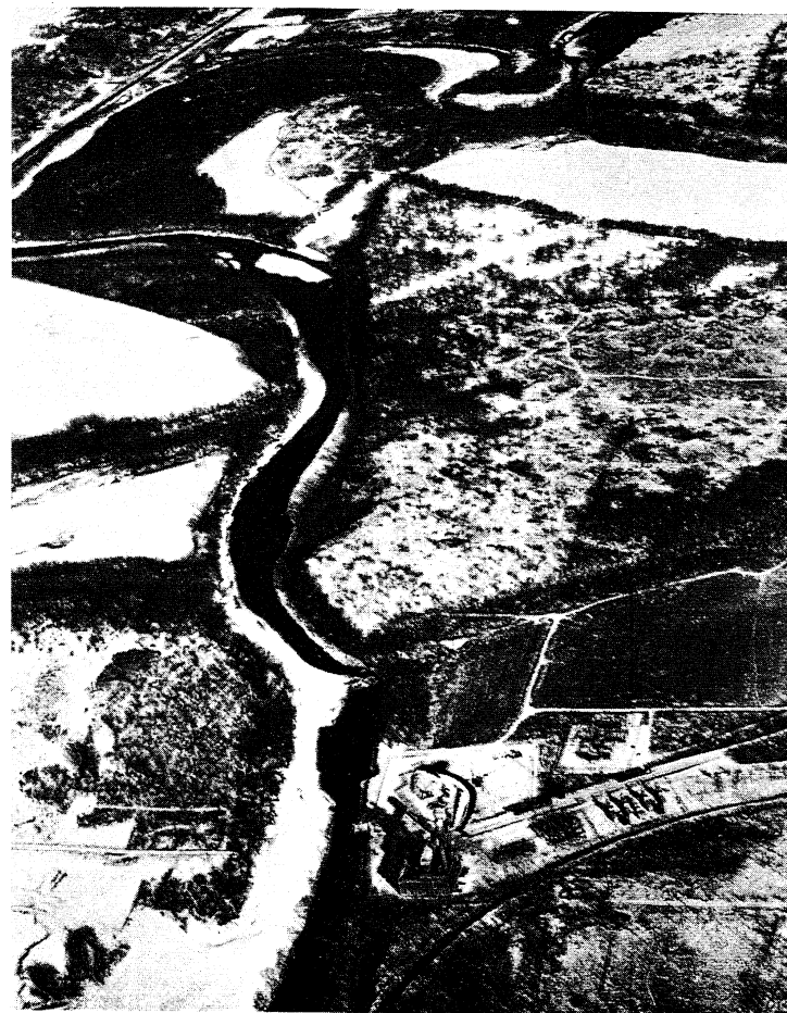
Fig. 29 - Aerial View of Minnesota River Looking Downstream from Wilmarth Power Plant at Mankato - February 16, 1974
