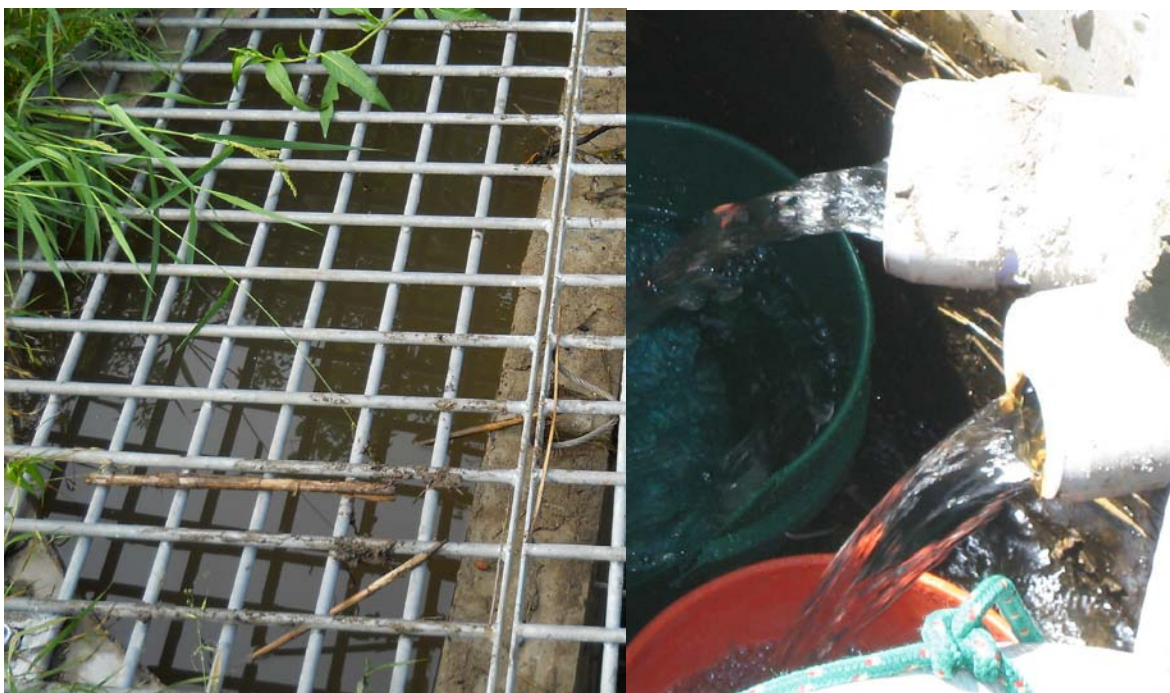
Figure 5: Water clarity within the pond (left, shown in the outlet structure) and after treatment by the iron-enhanced filtration trenches (right, shown at the effluent of the underdrains).
