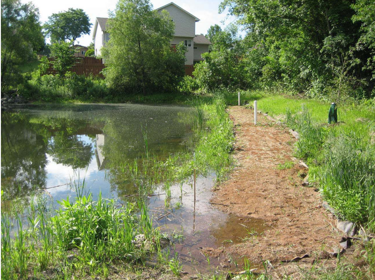
Figure 2: Pond 1 with iron enhanced filtration trenches in Prior Lake, MN
