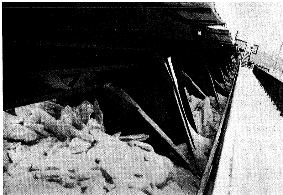
Fig. 12(b). Ice jam breaking through the Coon Rapids Dam in December 1984.
