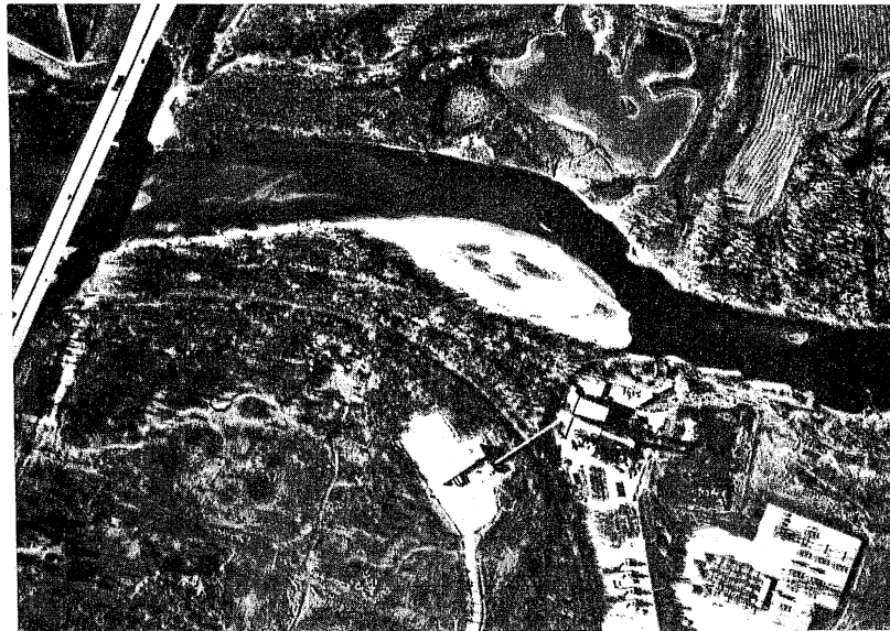
Fig. 14b. The exposed bar upstream of the intake at 5,000 cfs in the prototype.
