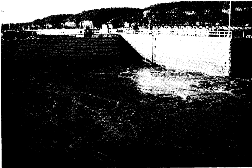
Fig. V-3. Discharge from operational lock.
