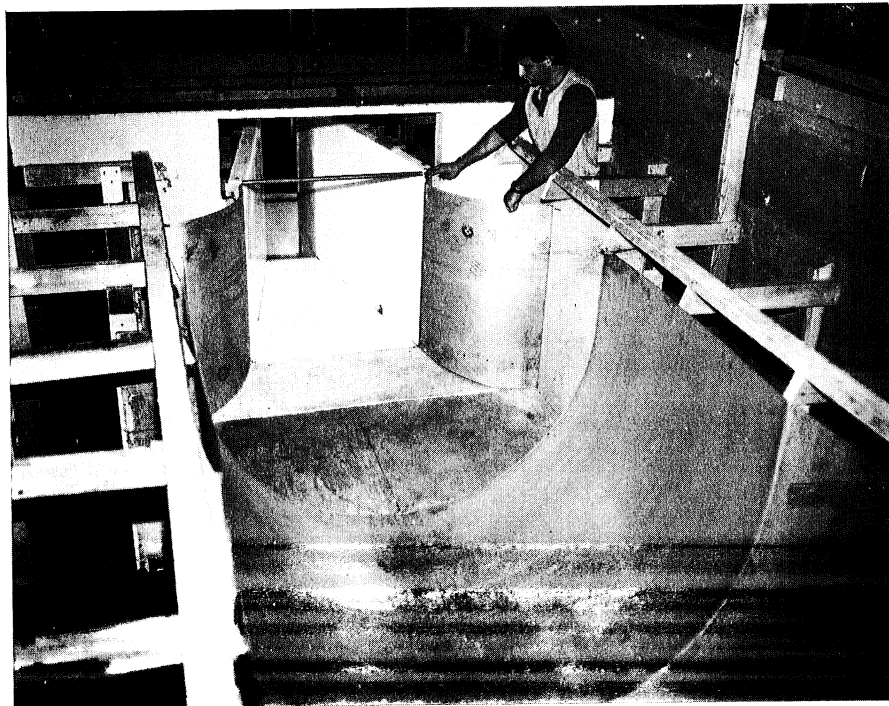
Photo 10 - Type B2. The 5-ft diameter inlet channel.
