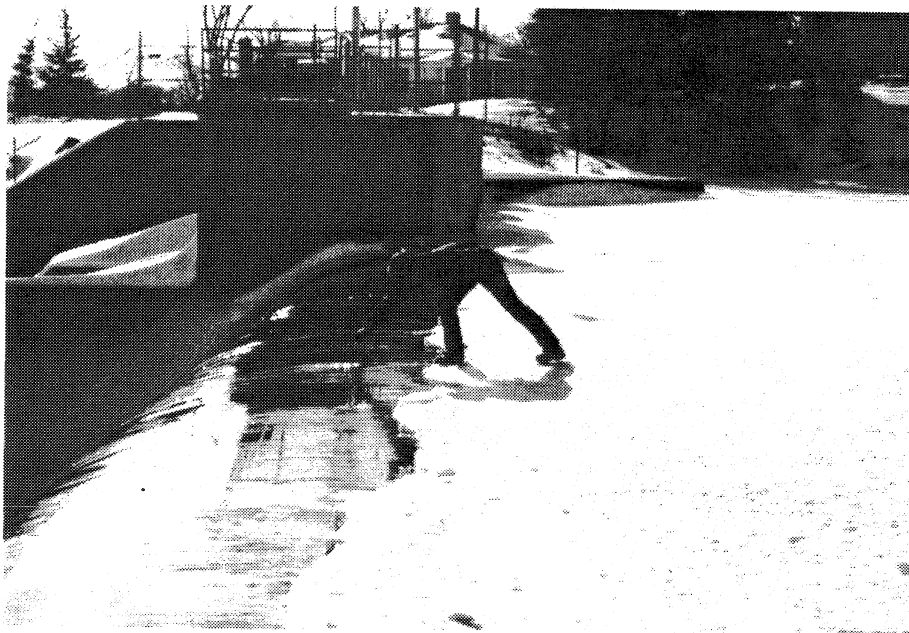
Photo V-4. Elk River Dam, January 10, 1986, location F2 upstream sampling. Note: The jagged ice edge the result of ice clearing from spillway crest.
