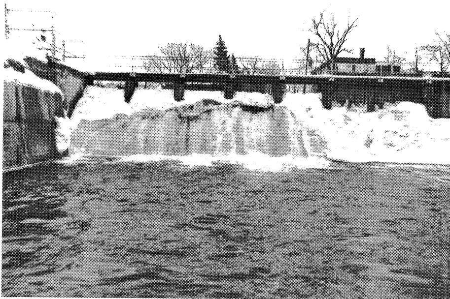
Photo X-1. New Richmond Dam, February 19, 1985; discharge characteristics.
