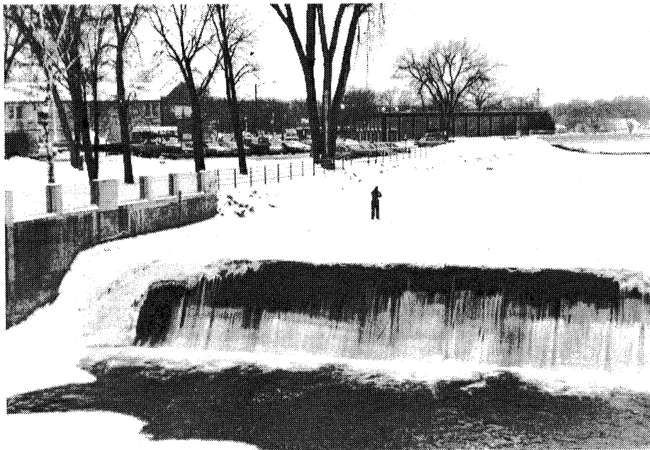
Photo XI-1. Northfield Dam, A1 sampling location. Note: the large variation of aerated flow due to the large portions of concrete removed by concrete spalling.
