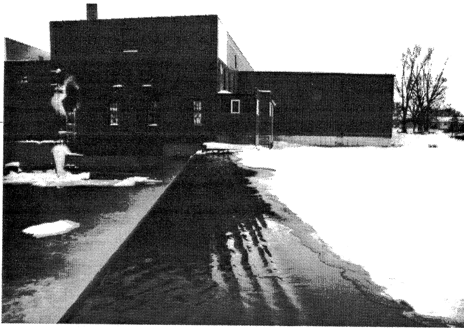
Photo VI-1. Faribault Woolen Mill Dam, December 17, 1985, upstream flow characteristics.
