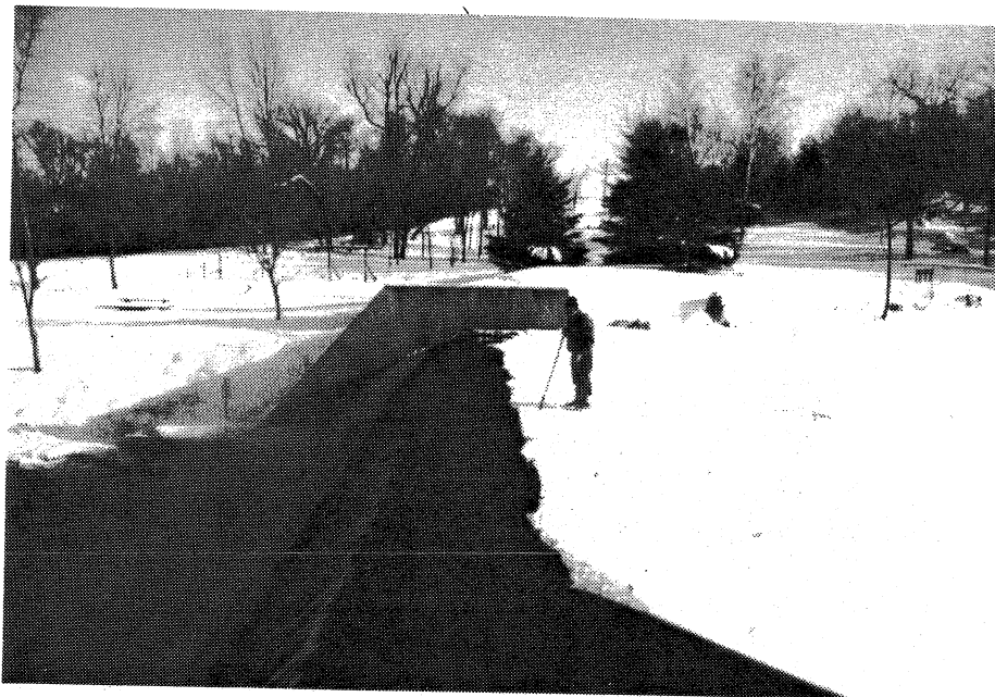
Photo II-4. Kost Dam, December 13, 1985, upstream ice formation after clearing with ice pick.
