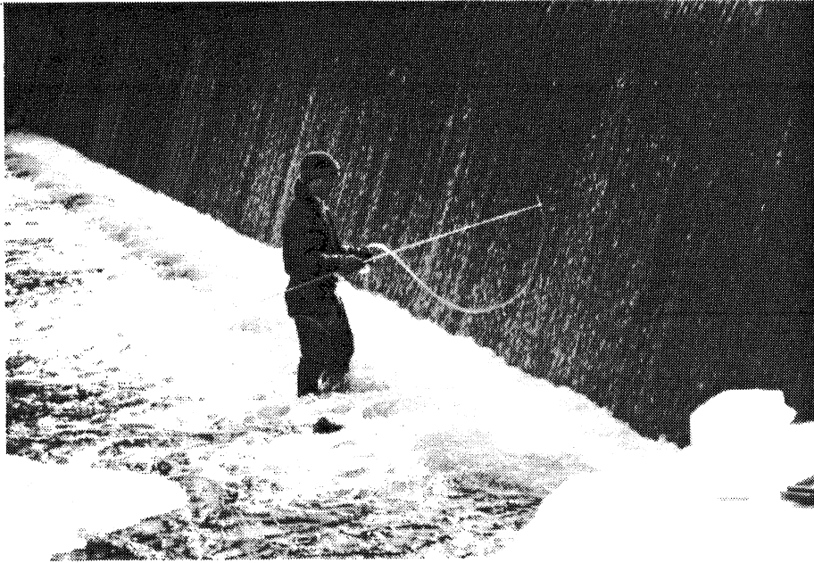
Photo VI-3. Faribault Woolen Mill Dam February 28, 1986, spillway aeration. Note: Spillway sampler in foregrounds.
