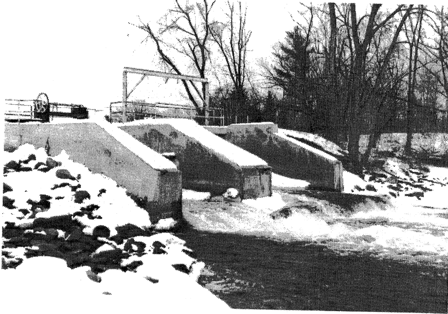
Photo VII-1. Flow leaving the Amery Dam tainter gate spillway.
