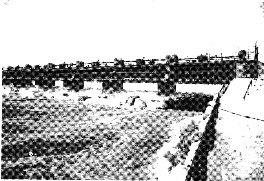
Photo VIII-2. Frazil ice jam tailwater increase, January 9, 1986.
