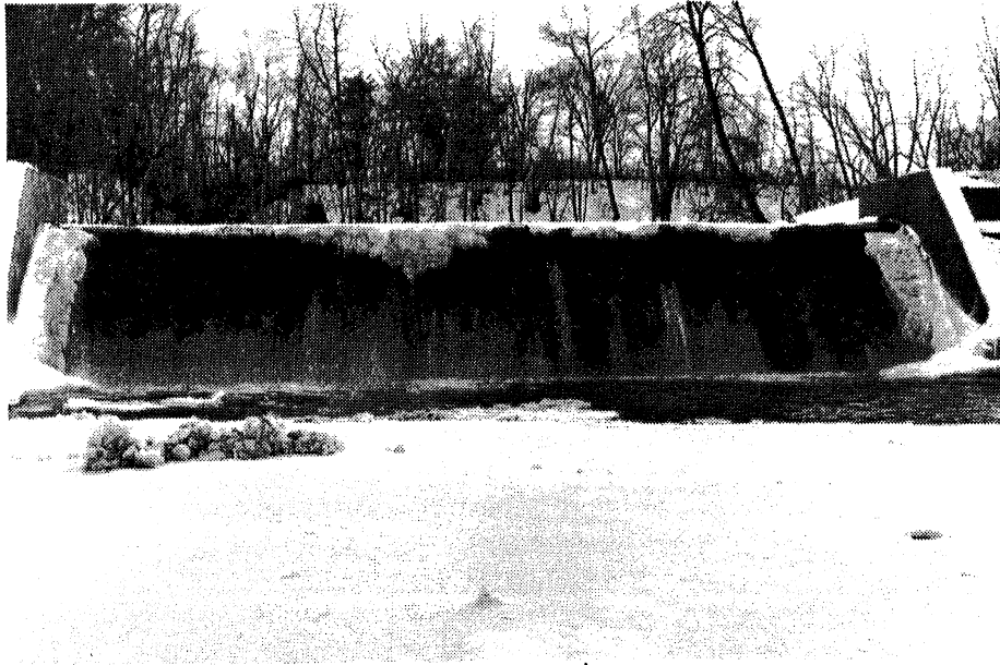
Photo II-1. Kost Dam, February 2, 1985, spillway face ice formation.
