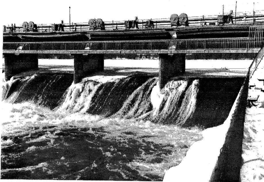
Photo VIII-1. Spillway crest ice caps, January 22, 1985.
