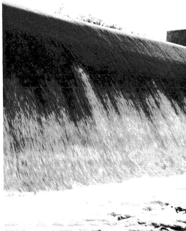
Photo II-10. Kost Dam, March 10, 1986, spillway aeration.
