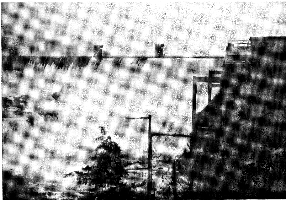
Photo XIV-2. Byllesby Dam, February 23, 1985, left rock spillway flow.
