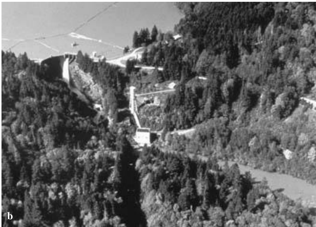
Figure 2.3. Aerial view of the two Elwha River dams and reservoirs. (a) Aerial view of Elwha Dam and Lake Aldwell (Source: http://www.nps.gov/archive/olym/elwha/photos/aeriallwr.htm ). (b) Aerial view of Glines Canyon Dam (Source: http://www.nps.gov/archive/olym/elwha/photos/aerialglines.htm ).
