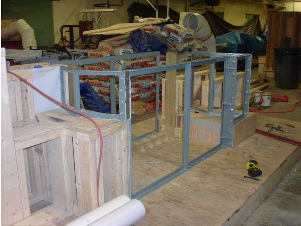
Figure 6. View of the model structure under construction.
