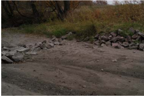
Figure 6.36 Sedimentation behind stream barb.
