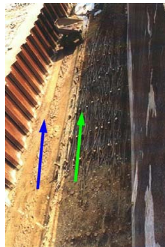
Figure 8.6 Fascine layer. All dimensions are in meters (1 m = 3.3 ft).
