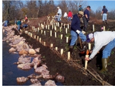
Figure 6.17 Stacking fascine at toe and placing stakes for brush mattress.
