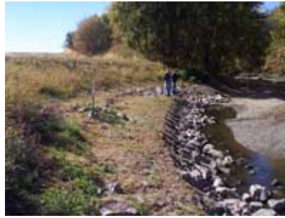
Figure 6.26 Sediment deposited on top of rock toe in upstream part of curve.
