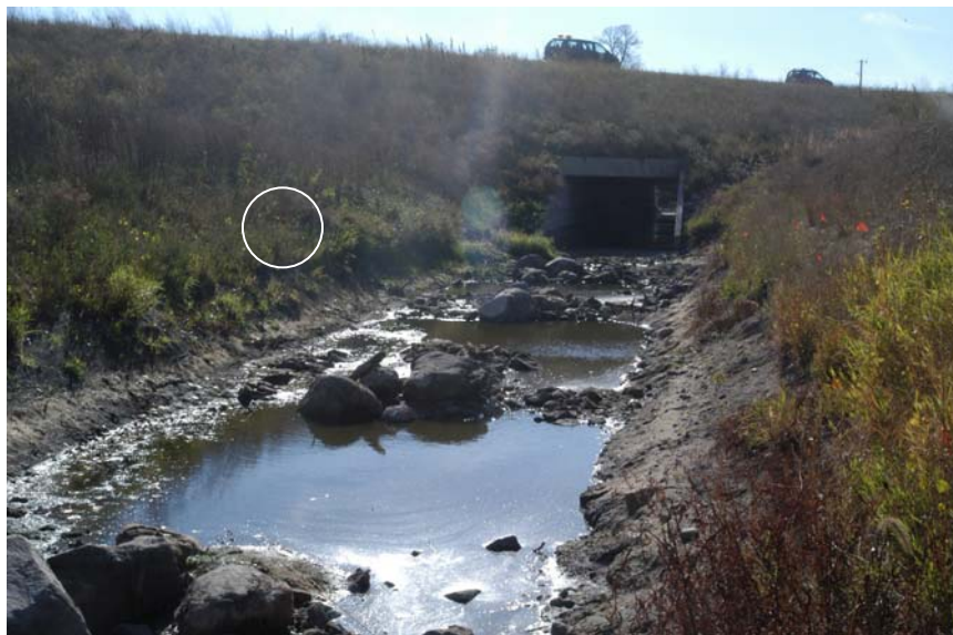
Figure 6.5 Another photo looking upstream. The white circle points out the area where there is a localized slumping of the bank. Runoff from the highway surface is directed into that area.
