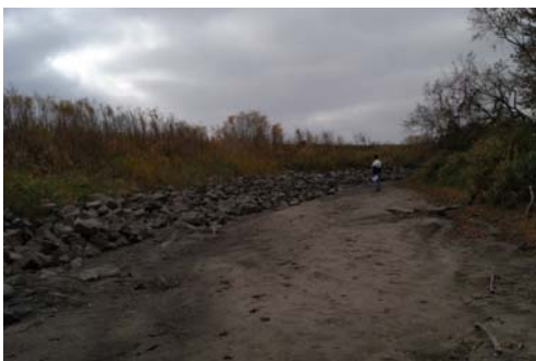
Figure 6.34 Entire channel. Note rocks from riprap in center of channel.
