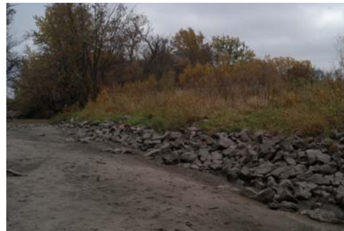
Figure 6.31 Fascine area, looking downstream.
