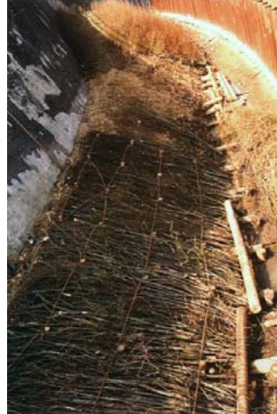
Figure 8.4 Brush mattress with willows. All dimensions are in meters (1 m = 3.3 ft).
