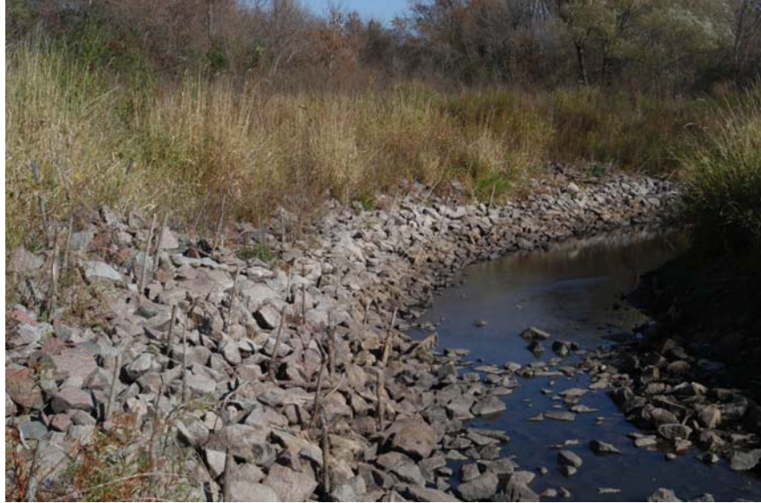
Figure 6.4 Dead willow posts in the riprap.
