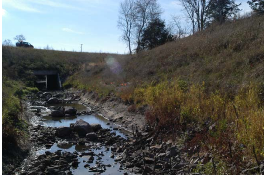
Figure 6.2 Same reach of the stream, but looking back at the culvert. The bank on the right side is showing signs of instability.
