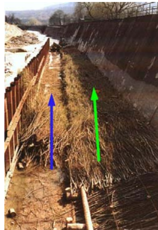
Figure 8.5 Branch layer. All dimensions are in meters (1 m = 3.3 ft).
