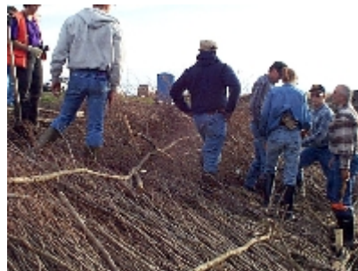
Figure 6.21 Brush mattresses with log anchors.
