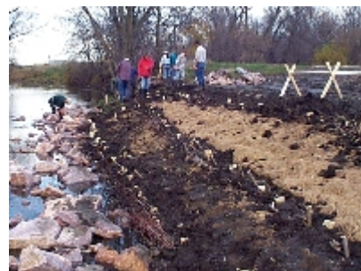
Figure 6.15 View of finished horizontal fascines in foreground and diagonal fascines in background by people.
