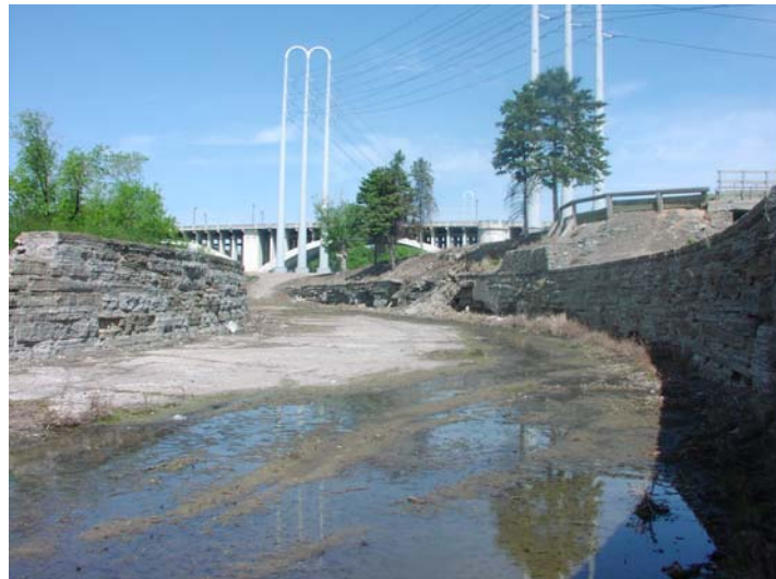
Figure 8.14 Wasteway no. 1: View from downstream looking upstream.
