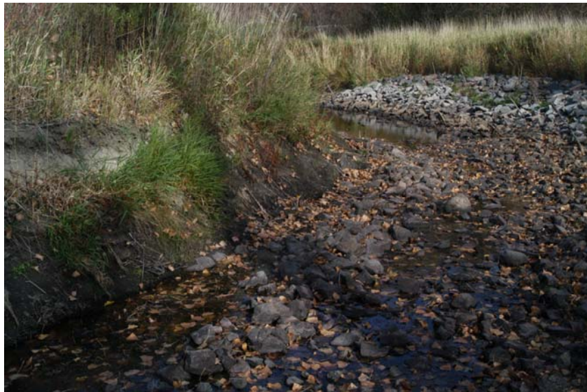
Figure 6.3 A bank where it can be seen that the riprap is no longer on the bank. Either the bank has eroded from behind the riprap or the rocks were carried downstream from the upstream bend where riprap was placed.
