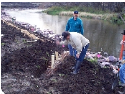
Figure 6.14 Installing diagonal fascines.
