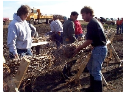
Figure 6.11 Frame used to construct fascines on site; made of 2x4's.
