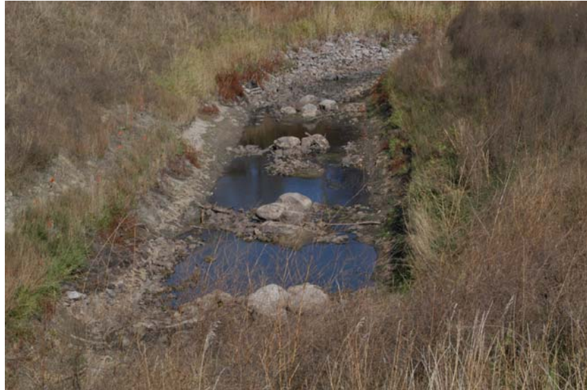
Figure 6.1 The reach initially downstream of the culvert under TH-12. Erosion on the banks can be noted, along in-stream structures that were placed in the stream.
