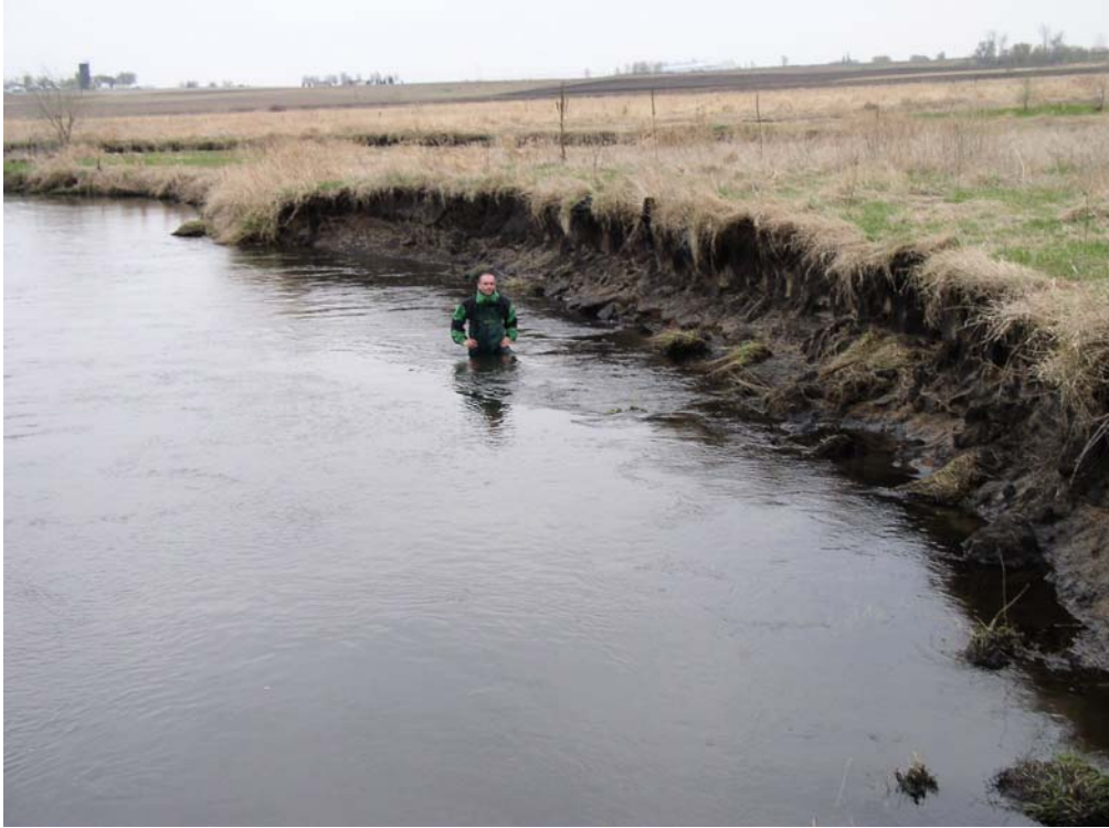
Figure 8.23 Bank erosion along a bend
