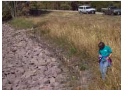
Figure 6.27 Soil washed from techniques immediately above the rock toe.
