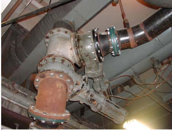
Figure 3.4. 24-inch tap from supply channel, 12-inch pipe and Tee to Pipe B (upper right) and Pipe A (bottom left). Note hydraulic-actuated gate valves on each pipe for control of flow rates.
