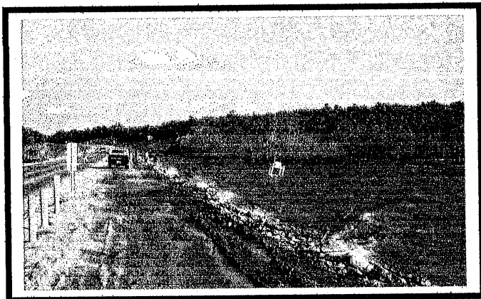
Figure 2-3 - Station DL2 located west and south of the Highway 20 bridge.
