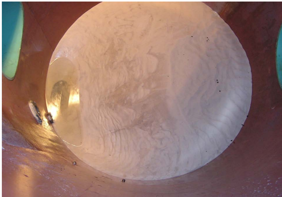
Figure 3.14. Overhead View of the Sediment Deposit in the Sump after a Washout Test. Inflow during the Test Was from Right to Left
