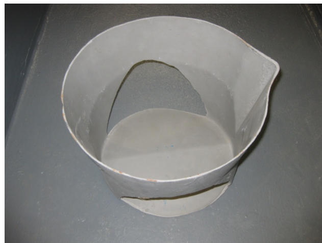
Figure A-13: Stormceptor drop tee
