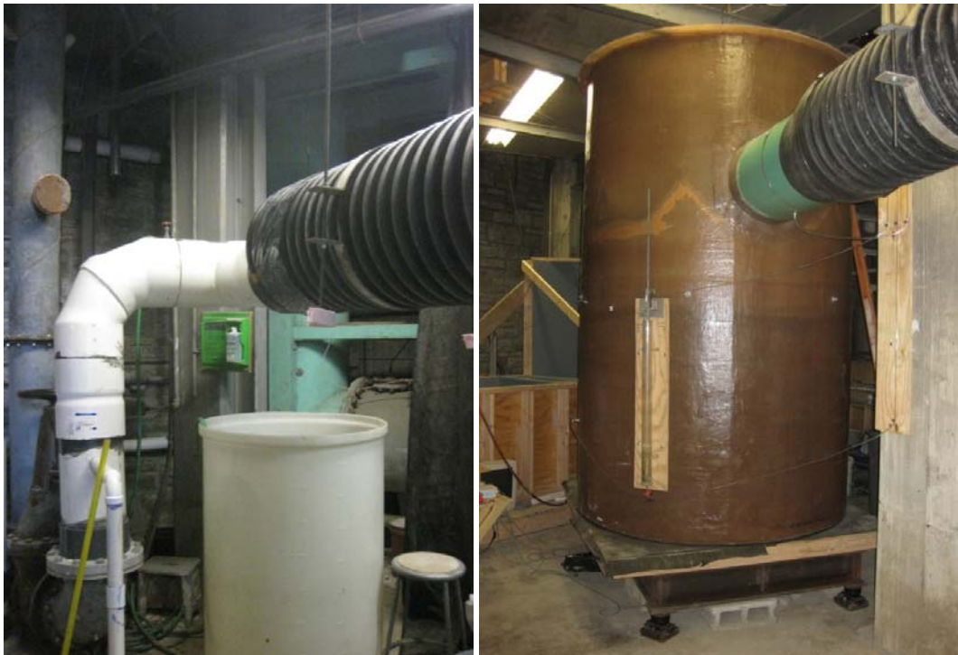
Figure A-11: Stormceptor water feed piping
