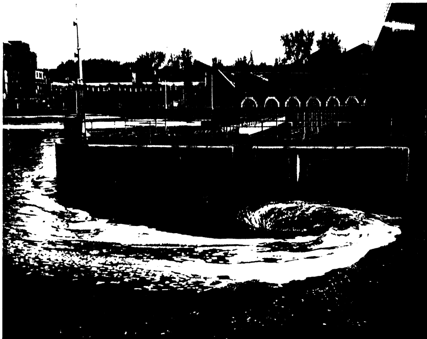
Photo 2. View showing vortex in conjunction with the front bullnose pier at intake No. 1, Lower St. Anthony Falls Lock and Dam.
