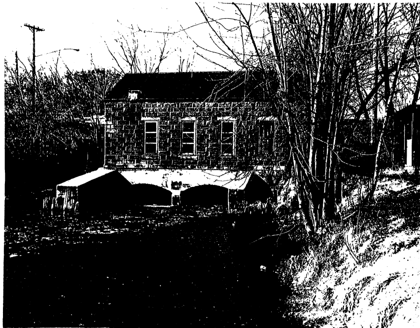
Fig. 9. Park Rapids hydropower plant. View from downstream.
