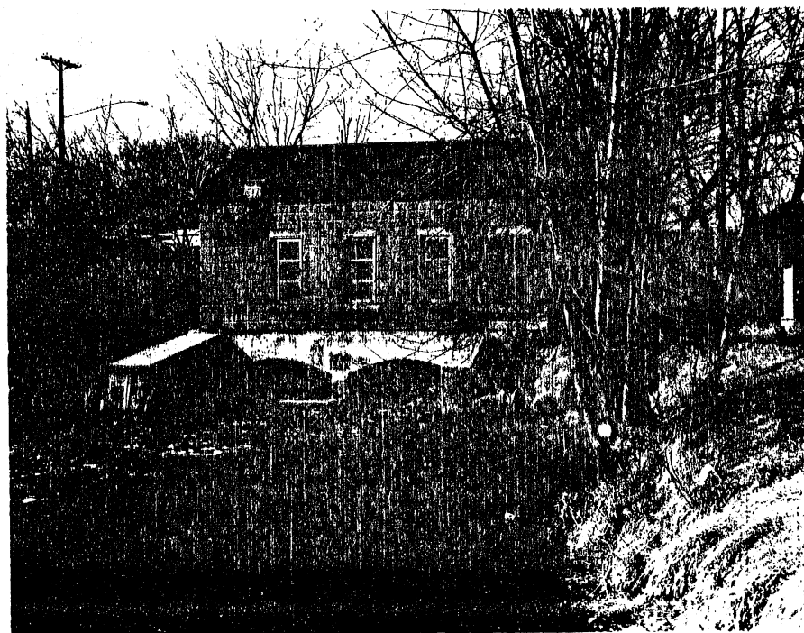
Photo 2. View from downstream of generator room and powerhouse outlet with wingwalls.
