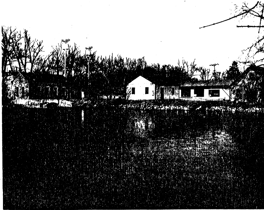
Photo 5. View from tailwater pool of powerhouse and the three Minnesota DNR fish hatchery buildings.
