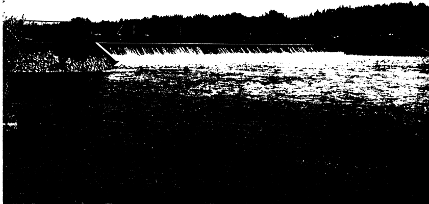
Fig. 5. View from Right Bank Showing Unregulated Ogee Spillway and 10th Street Bridge in Background.
