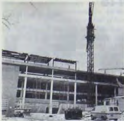
Construction well underway on new Law School building on Minneapolis West Bank campus.
