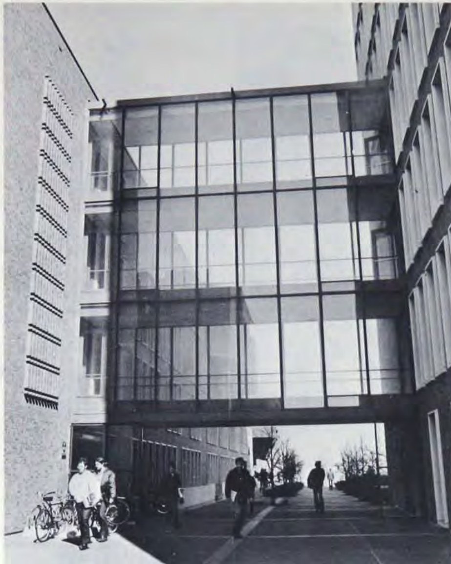
THIS THREE-TIERED, enclosed pedestrian walkway between Blegen Hall and the Social Sciences Tower on the West Bank campus of the University of Minnesota will receive heavy use during the winter quarter months.
