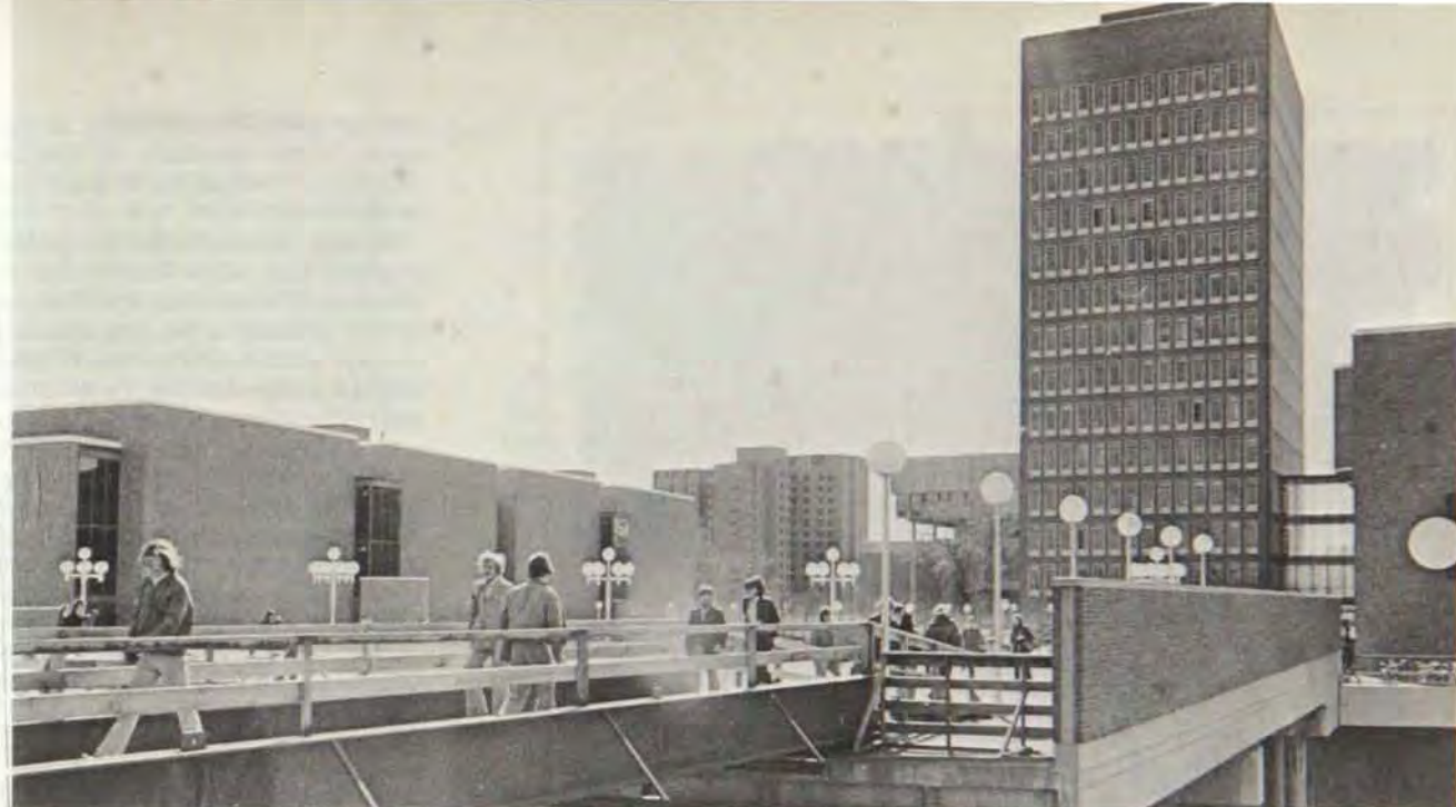
TODAY THE COLLEGE of Liberal Arts is far-flung, with classrooms on both the East and West Banks of the University. On the West Bank, many of these are in the Social Sciences Tower, which is the tallest building in the photo above. To the left of the tower, is a classroom building, Middlebrook Hall (a residence hall) and a portion of the Rarig Center for the Performing Arts. To the right of the Social Science Tower is a portion of Blegen Hall, which also is the site of some liberal arts instruction.
