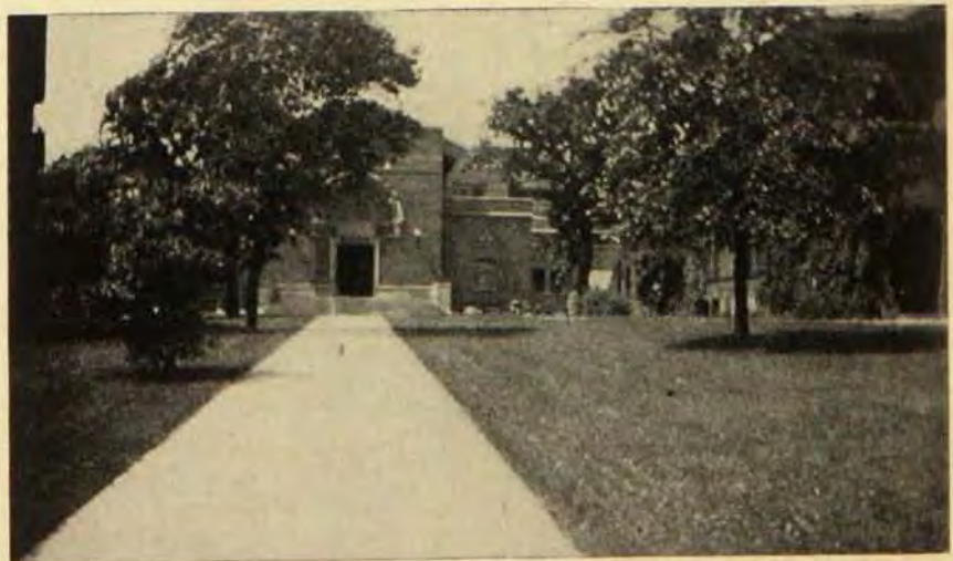
Entrance to women's gymnasium
