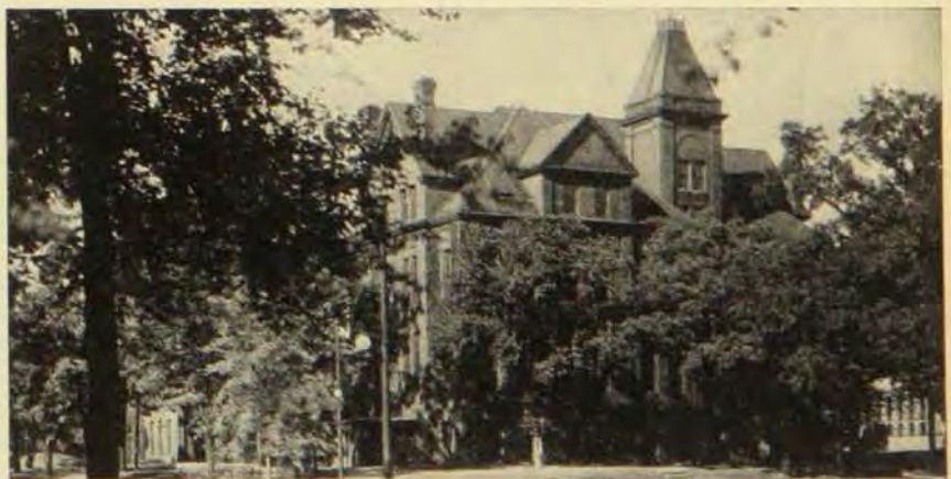
Business School students this week celebrated the fact that a new building will soon replace this structure as the home of the School of Business Administration.
