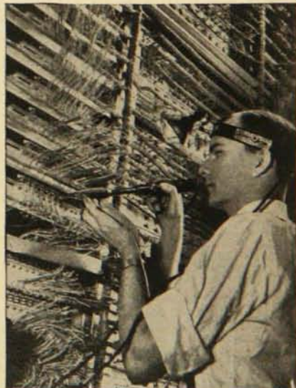
This skilled worker is performing a delicate operation on equipment for a new telephone exchange. He joins thousands of wires that will carry your voice wherever there are telephones.
