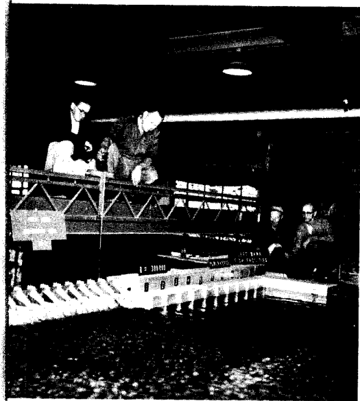
This is a scale model of the Priest Rapids project on the Columbia River, Washington, one of many project models planned and built by Laboratory personnel. Models are used for tests preliminary to actual construction at the site.
