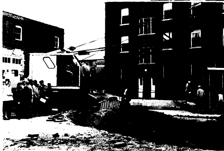
Ground Breaking for the VFW Cancer Research Center
