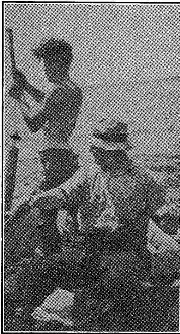
In the upper picture is shown the outfit of two canoes lashed together with a platform between, from which the depths of Minnesota lakes were dredged; below a deep-sea thermometer is shown being brought up from a hole 240 feet deep in Canadian waters of Lake Saganaga.
