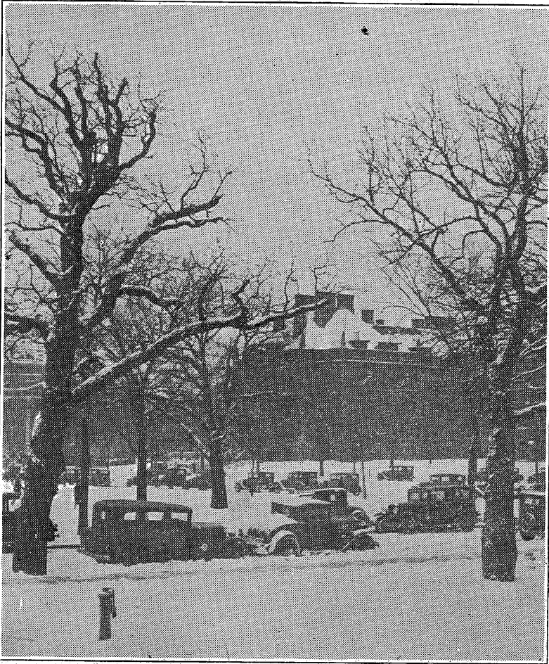
FOLWELL HALL, the principal recitation building, is shown in the distance, across the central campus east of the Knoll.
