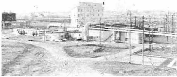
Fig. 10. Aerial view of continuous flow facilities (Bldg 302) RAL.
