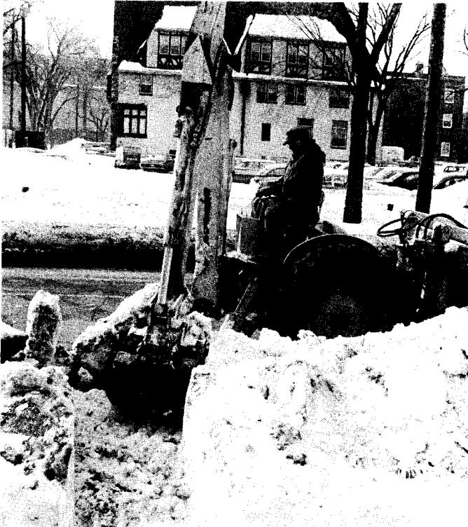
JIM HINES digs a trench with a Ford back-hole and front-end loader.
