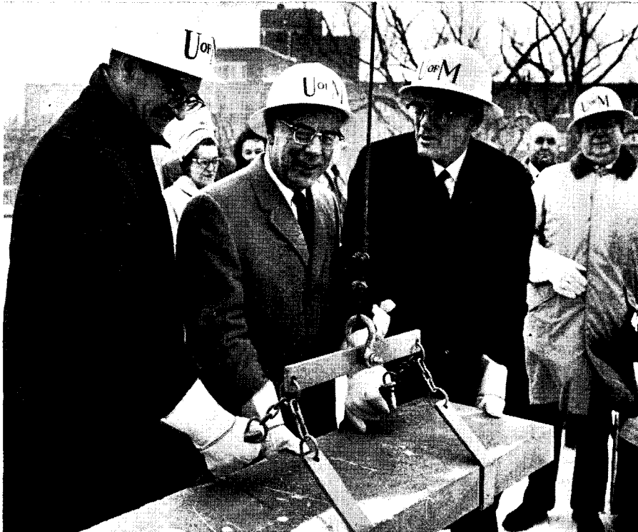
Dean Robert B. Howard, Campaign Manager Clyde E. Hegman, Masonic Past Grand Master Paul M. Olstad, and Vice President Laurence R. Lunden hoist a slab of limestone coping from the parapet of the Masonic Memorial Hospital roof. Construction of two additional floors will begin this spring with money raised by Minnesota Masons.
