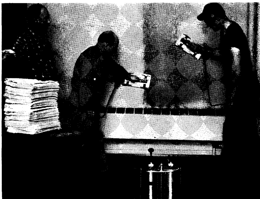
As William Stickels (l.) checks, Bryce Bunton rinses and Robert Mayberry washes a wall in basement of Pillsbury Hall. In foreground is water-tank,
