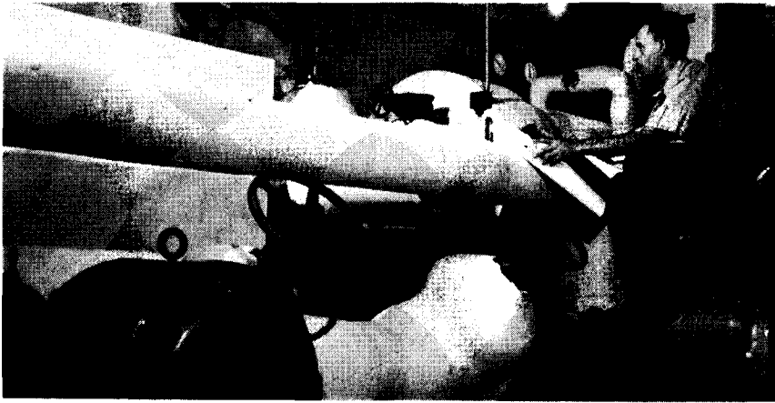
Nine miles of one-inch steel pipe encased in concrete are part of the Williams Arena ice-freezing mechanism. Don Veara supervises the equipment.
