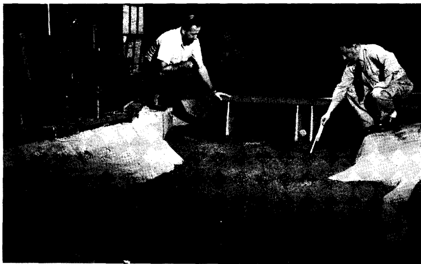
Above is a model of the Mississippi near the St. Paul High Bridge. The water has just been shut off, and the engineers are measuring movement of the river bottom. The engineers are Saul Fidelman, left, and Franklin Ryder.
