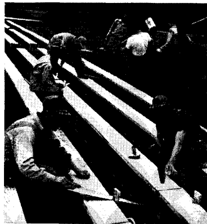
Carpenters construct benches for graduating class. In the foreground, left to right, they are Elmer Adelman, Harold Brown, Woodrow Carlson, and Ken Carlson.
