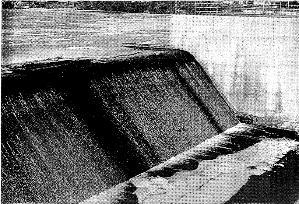
Photo VI-9 Spillway Elk River Dam
