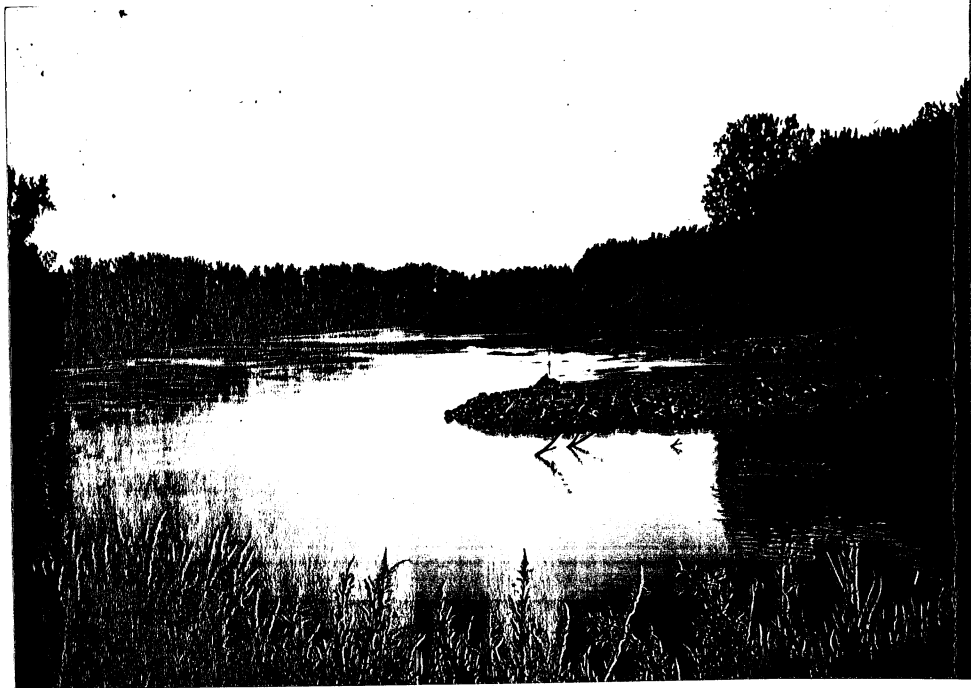
Figure 1.3 View of two of the rock spur dikes actually installed on the Minnesota River just upstream of the State Highway No. 93 bridge.
