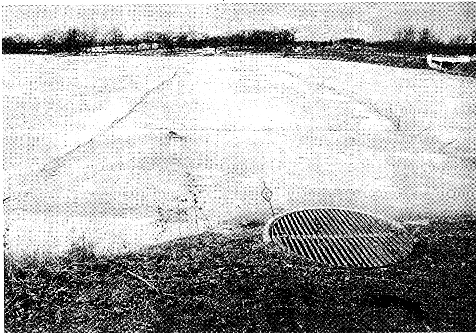
Photo 12. Area of ice above operating manifold/diffuser. Note: Absence of open water (March 15, 1991).
