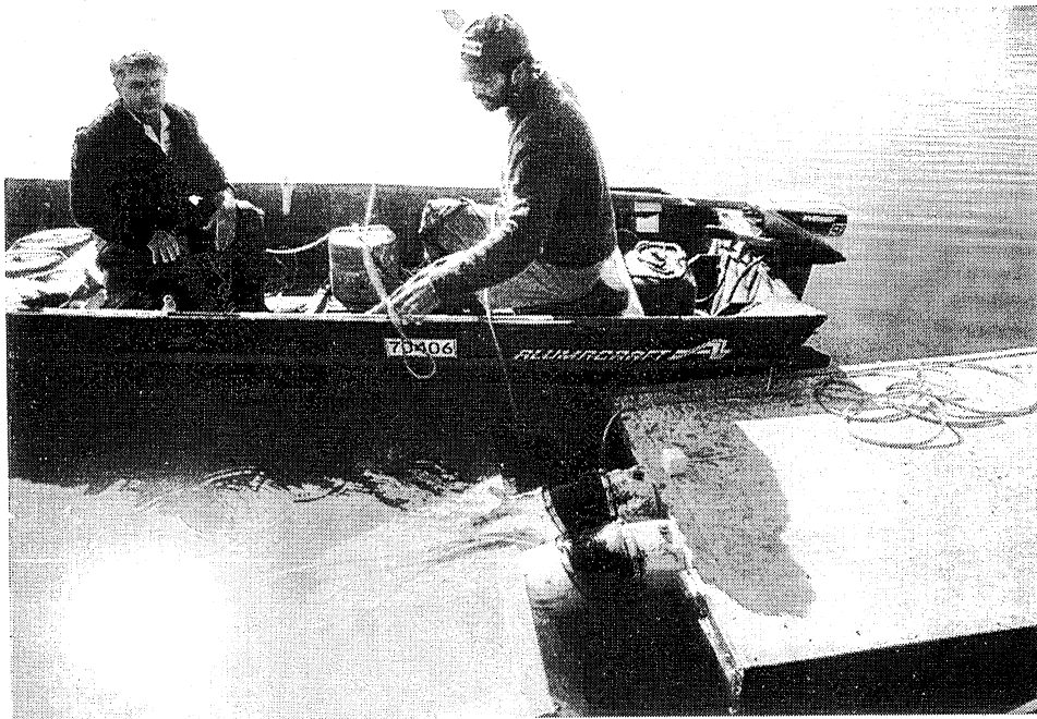
Photo 8. Attachment of anchors to and submergence of manifold/diffuser (Sept 1990).
