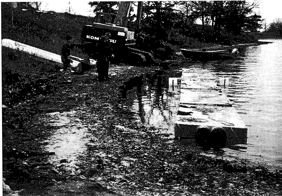
Photo 6. Manifold/diffuser (5 sections) connected and ready for installation (Nov 1989).
