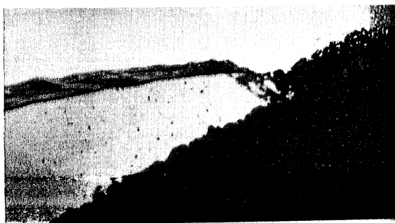
Wave Breaking on a Crushed-Rock Absorber
