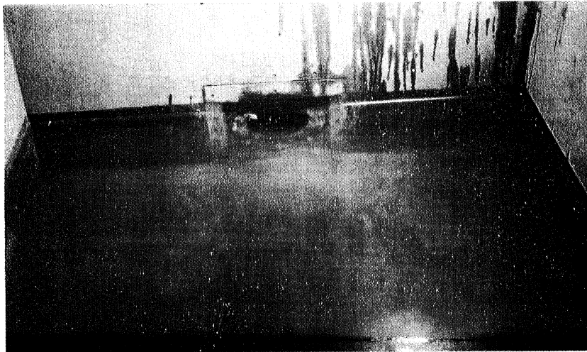
Fig. I-5 - Headwater Pool and Culvert Inlet
