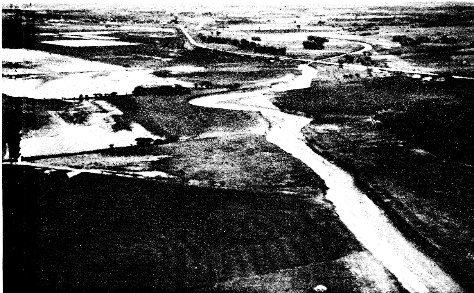
Fig. 2-8. Canal in Oklahoma showing meandering and secondary bank erosion. (Photo courtesy Dr. Don DeCoursey, ARS)
